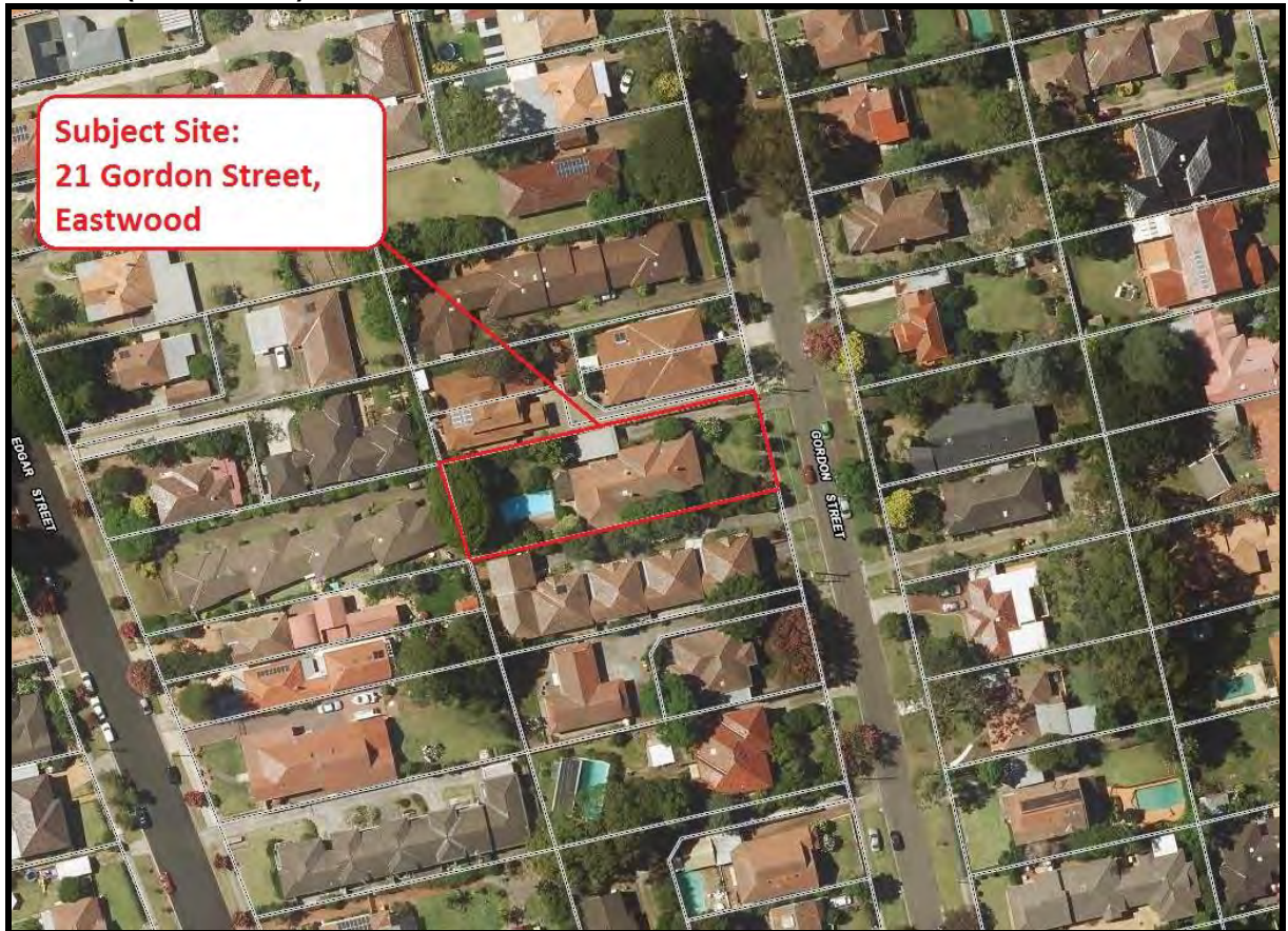
Figure 1: Aerial image of the subject site and surrounding development. Noted in this image is the prevalence of multi dwelling housing and dual occupancy development in the local area which is identifiable from the more expansive roof forms on select allotments.
