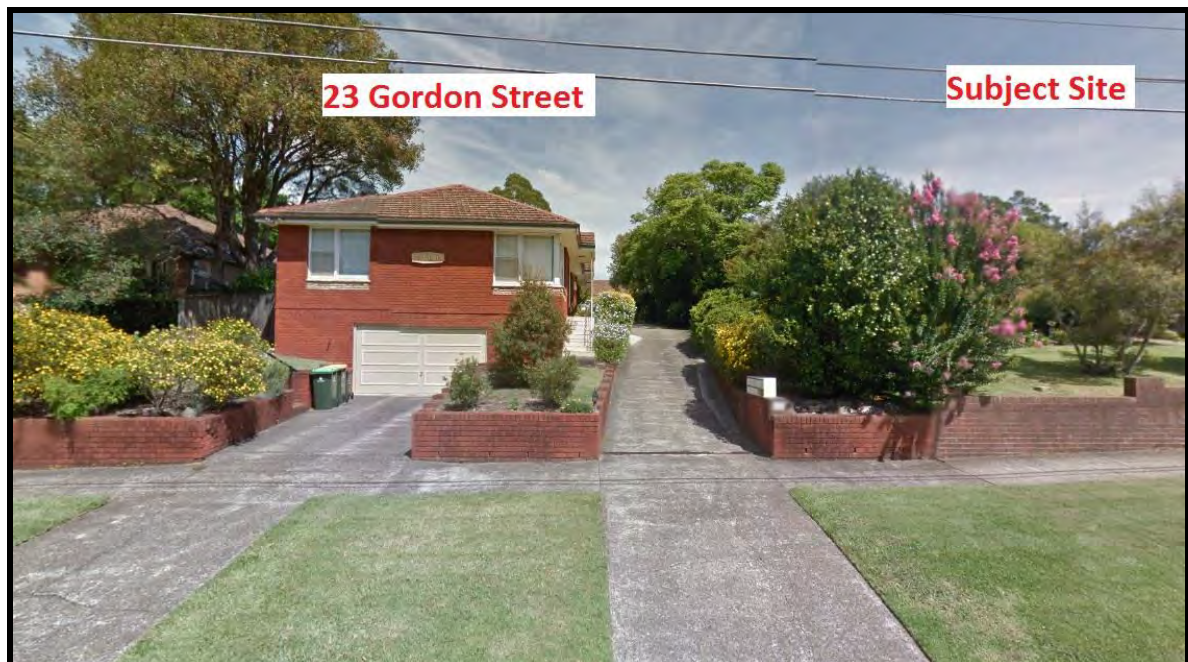
Figure 14. Photograph of the front of No. 23 Gordon Street with the subject site on the right. It can be seen in this image that the northern side No. 23 Gordon Street is dominated by the driveway. The development on the subject site proposed the driveway along the southern boundary meaning a substantial separation distance is provided between buildings, thus helping to minimise overshadowing impacts.
