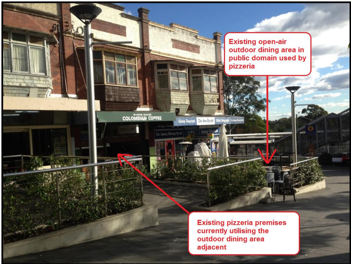
Figure 2: Photograph of subject site taken from the Constitution Road pedestrian plaza showing the location of the existing pizzeria premises and the existing open-air outdoor dining area adjacent to the pizzeria premises. Also noted in this image is the raised planter boxes which help delineate the outdoor dining area and the 2m wide pedestrian thoroughfare corridors that are located adjacent to each outdoor dining area.
