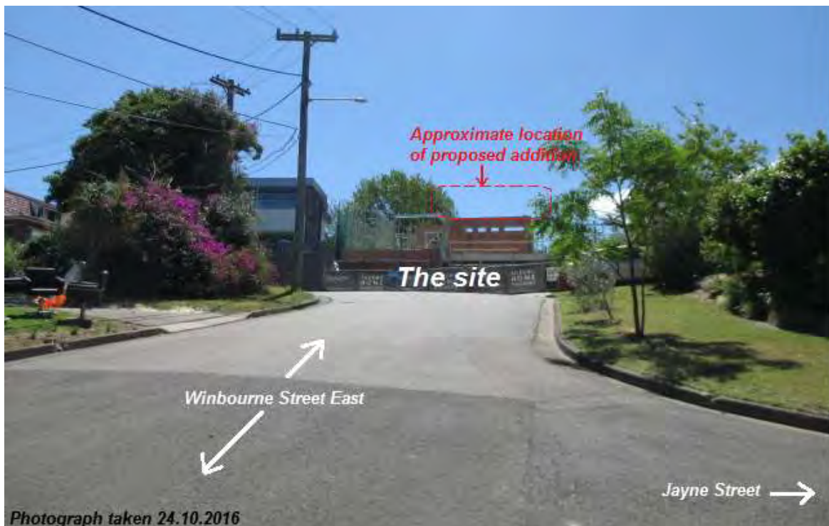
Figure 12. Photograph of site under construction showing approximate location of addition in the context of surrounding streetscape
