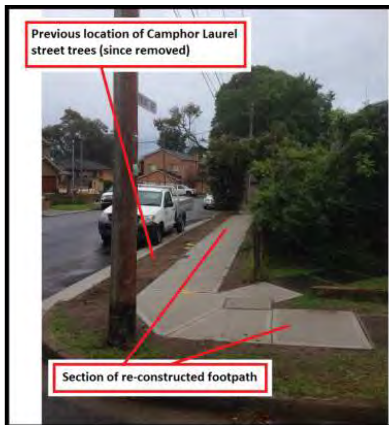
Photo (October 2016) showing footpath works already undertaken in Clermont Ave (front of No 9), including re-construction of footpath and removal of Camphor Laurel trees.
