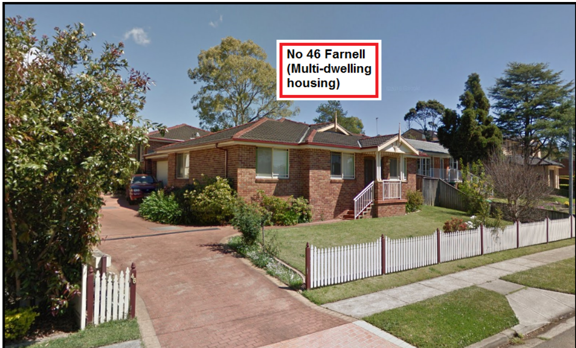
Figure 11. Multi-dwelling housing development at No 46 Farnell Street (approx. 150m south of the subject site) Source: Google Street View
