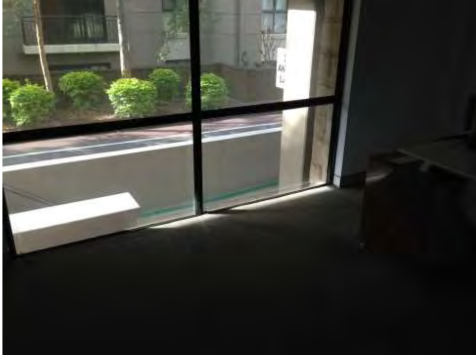
Left wintergarden window taken at 9.45am 21 June demonstrating the lack of sunlight penetration into the space.
