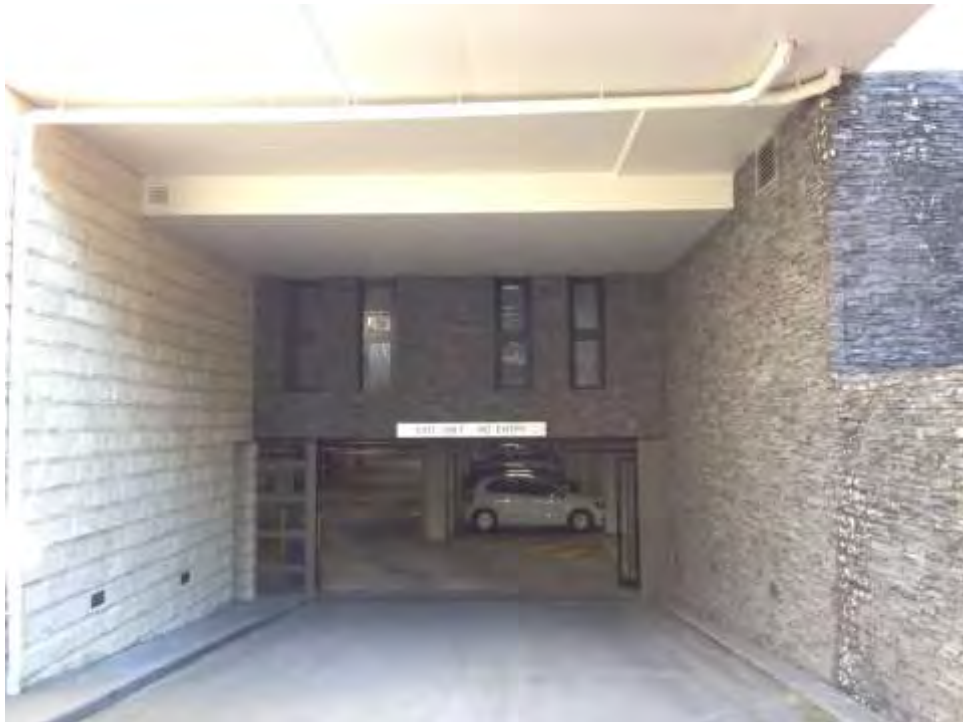
Photograph showing the windows to proposed Bedroom 1 and 2 located immediately above the car park roller door.
