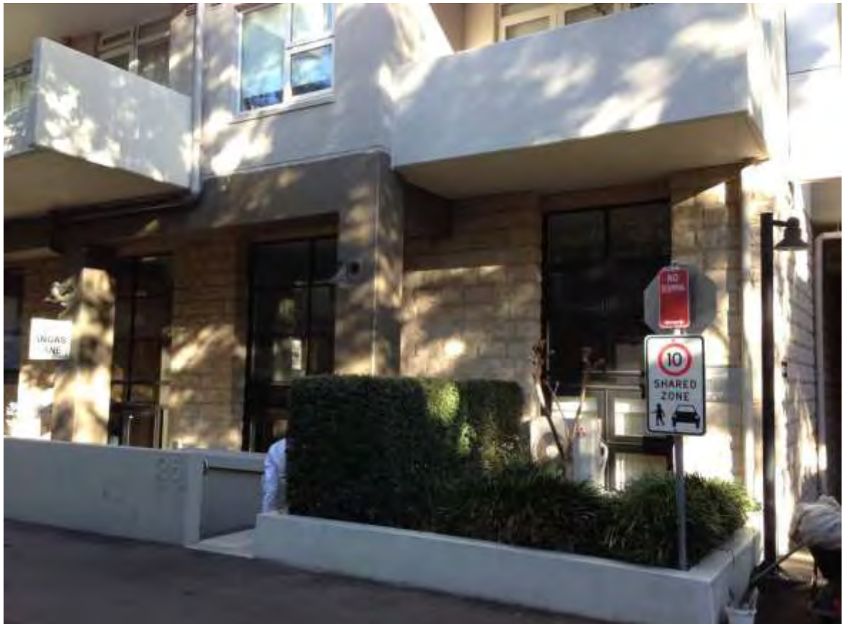
Suite 102 from the Angas Street frontage. Source: CPS site inspection photo, 21 June 2017
