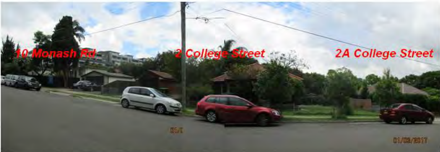
Figure 12. North east elevation – Photograph of existing site
