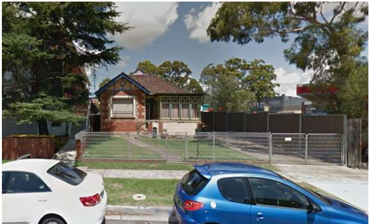
Figure 2: Subject site with existing dwelling house to be demolished.
