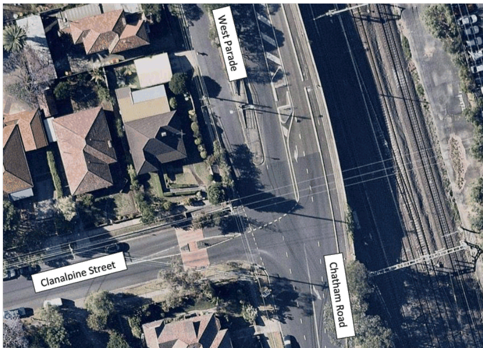
Figure 17: Intersection of West Parade/Chatham Road/Clanalpine Street
