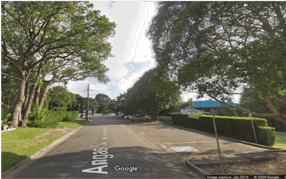
Figure 3: Street view of 90 Degree Indented Parking Area in Angus Street
