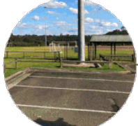
Existing car park
