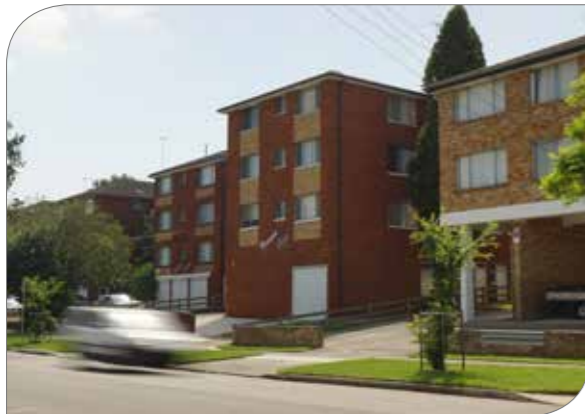
Typical 3 to 4-storey walk-up flat buildings located adjacent to the Town Centre. Many of these sites are in strata title and less likely to amalgamate.
