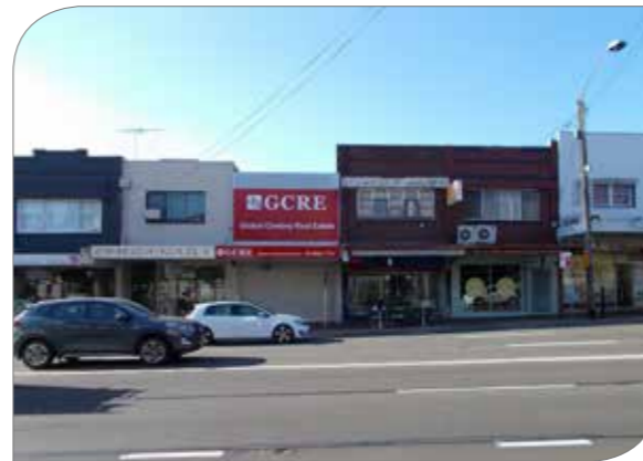
Typical 2-storey small shops on either side of Victoria Road
