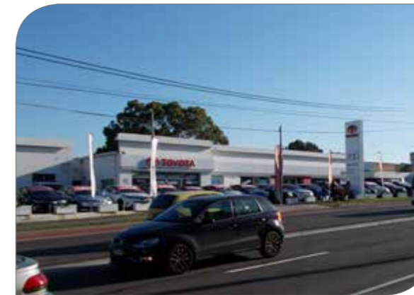
Typical low-scale commercial sites on Victoria Road. Many of these sites are large consolidated sites with the potential for redevelopment.
