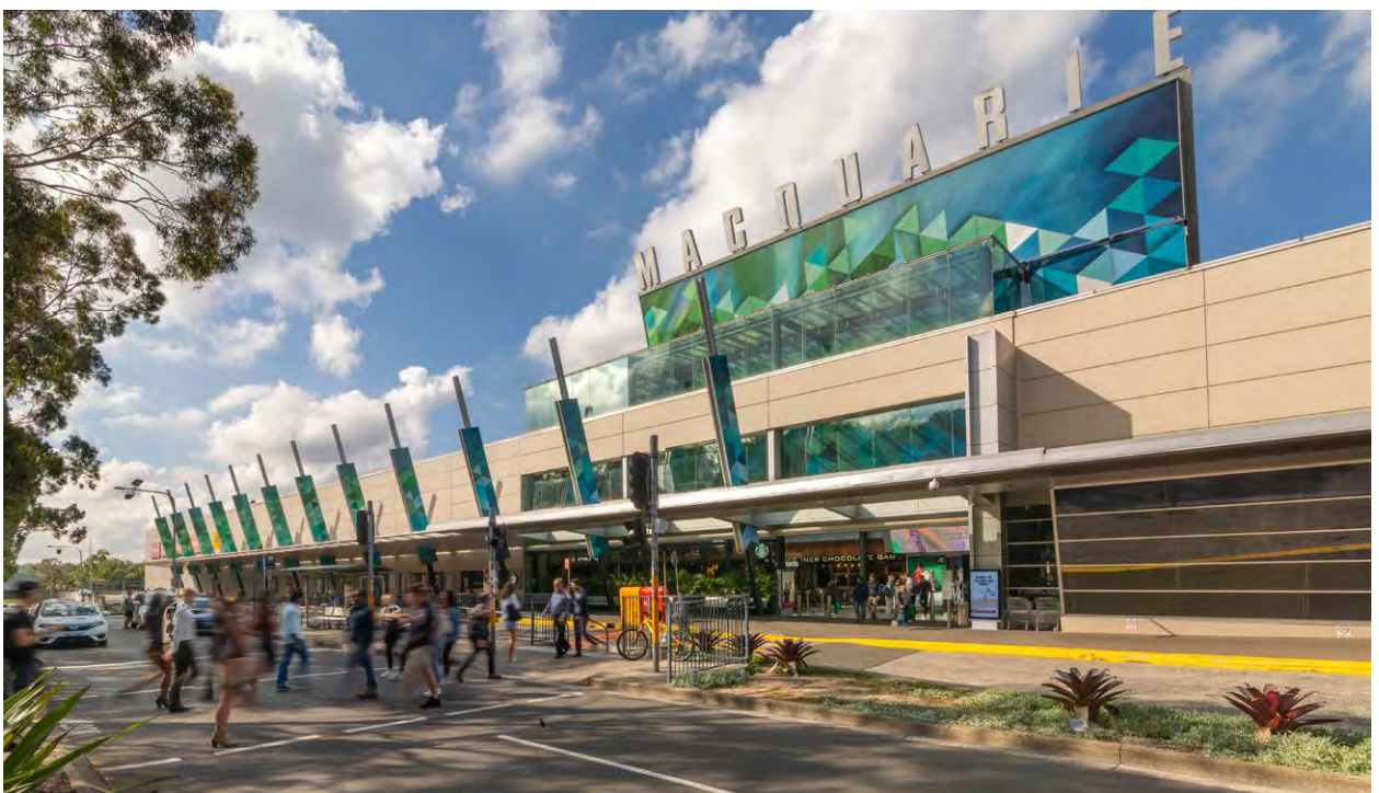
Macquarie Centre pedestrian entry
