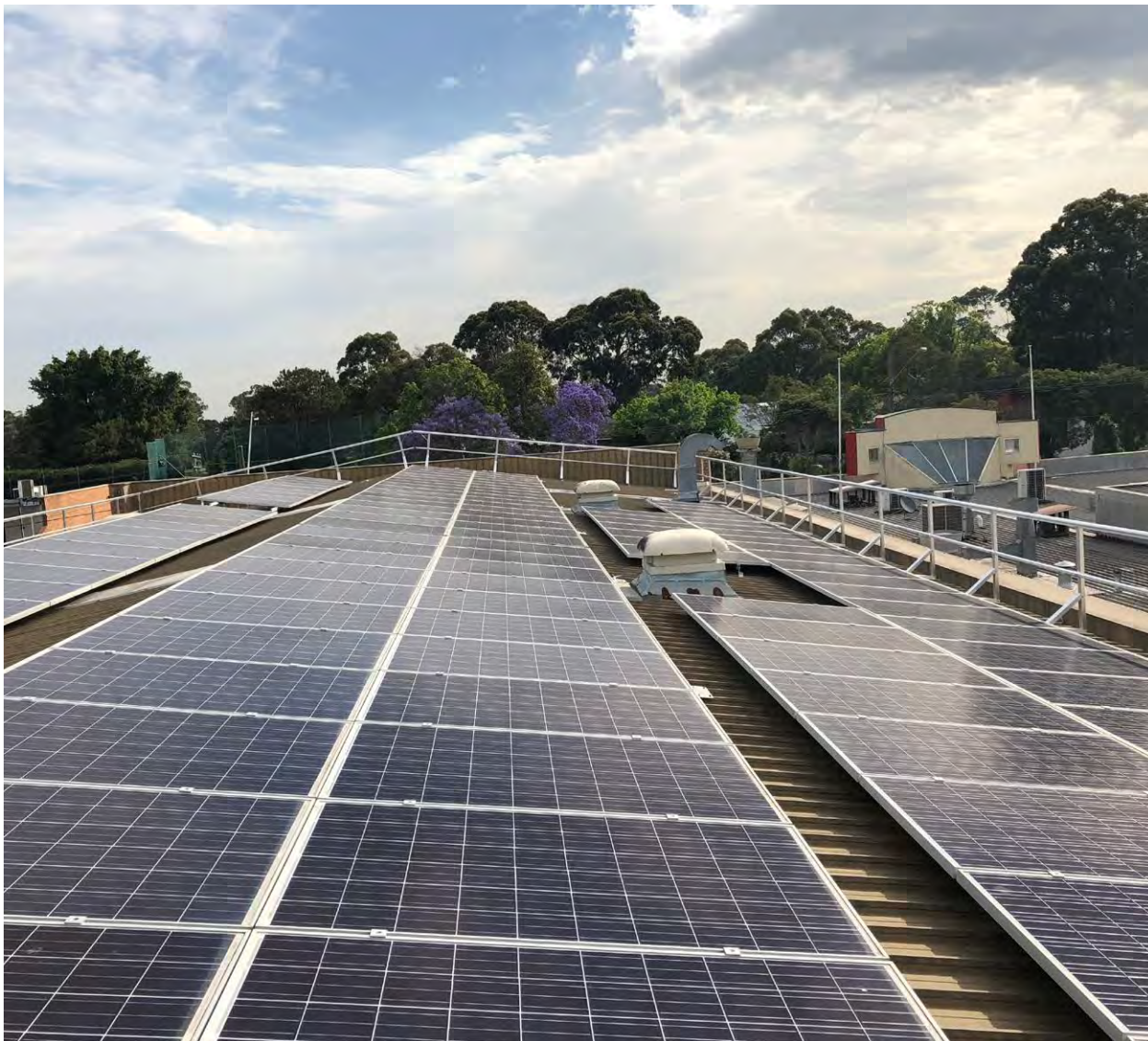
Solar panels on North Ryde Community Library
