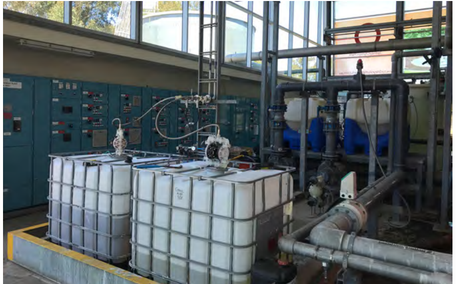
Pictured: Water recycling facility
