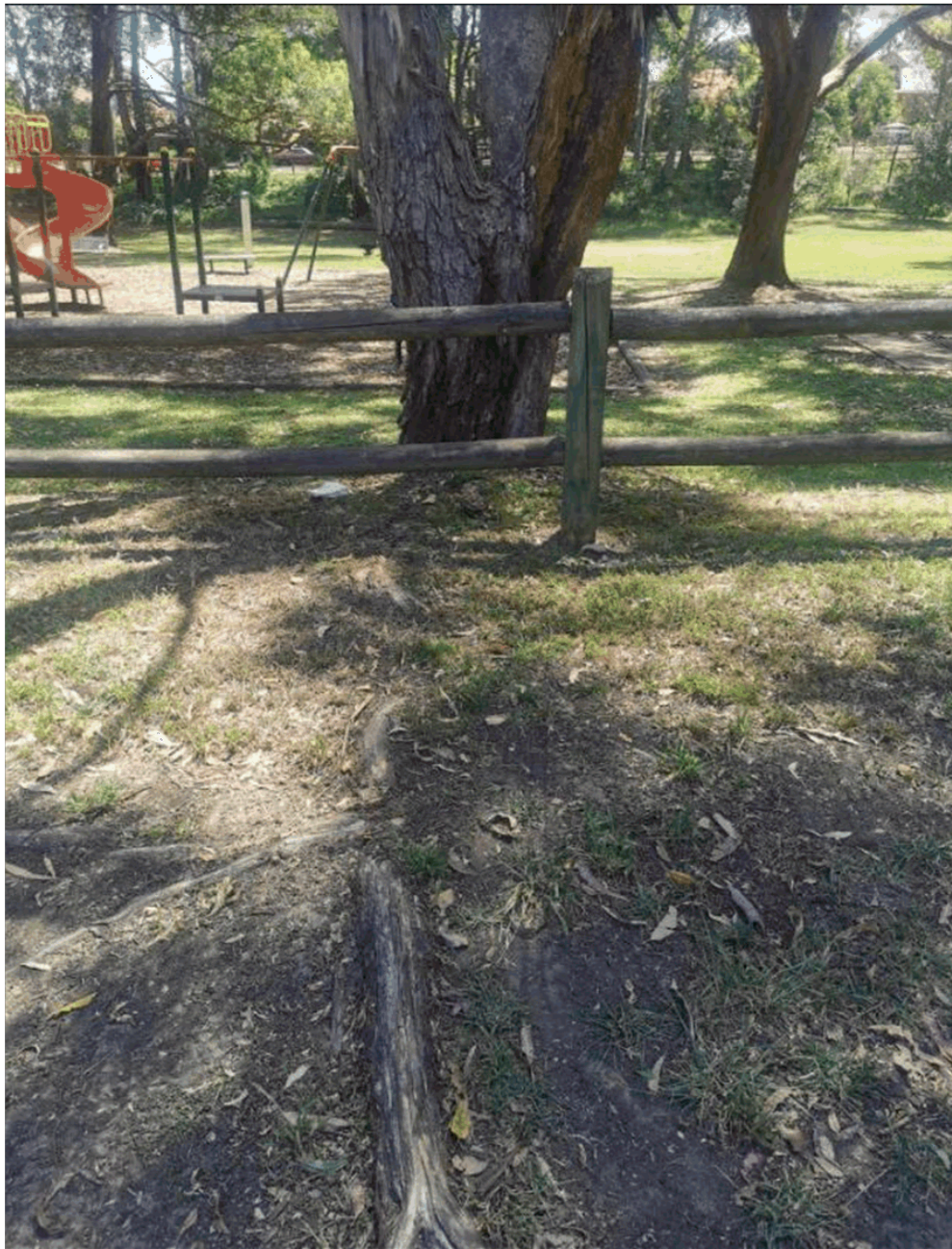
Figure 10- Large damaged surface root from tree #29.
