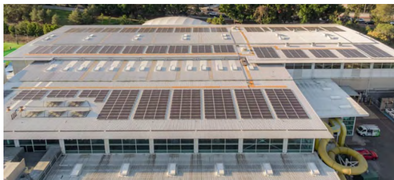
Image 17: Existing rooftop solar grid at Ryde Aquatic Leisure Centre
