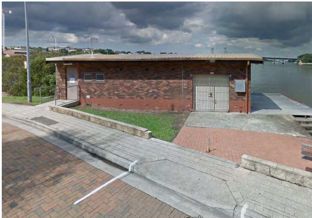
Image 2: Epping Scout Building 2008
