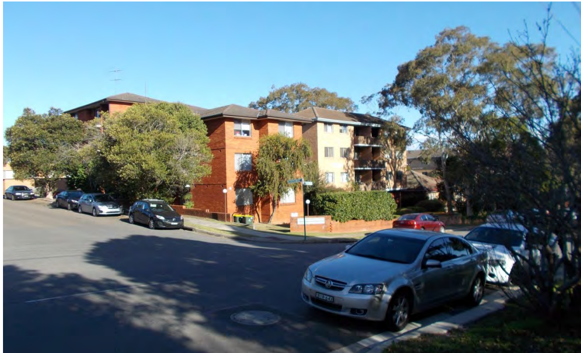
Figure 9. Existing residential flat buildings on the opposite side of Terry Road, viewed from the corner of Terry Road and Orchard Street
