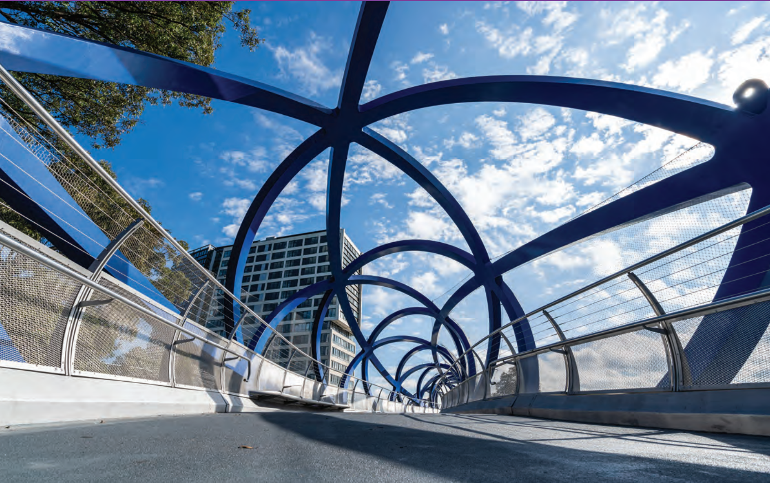
Footbridge at North Ryde.
