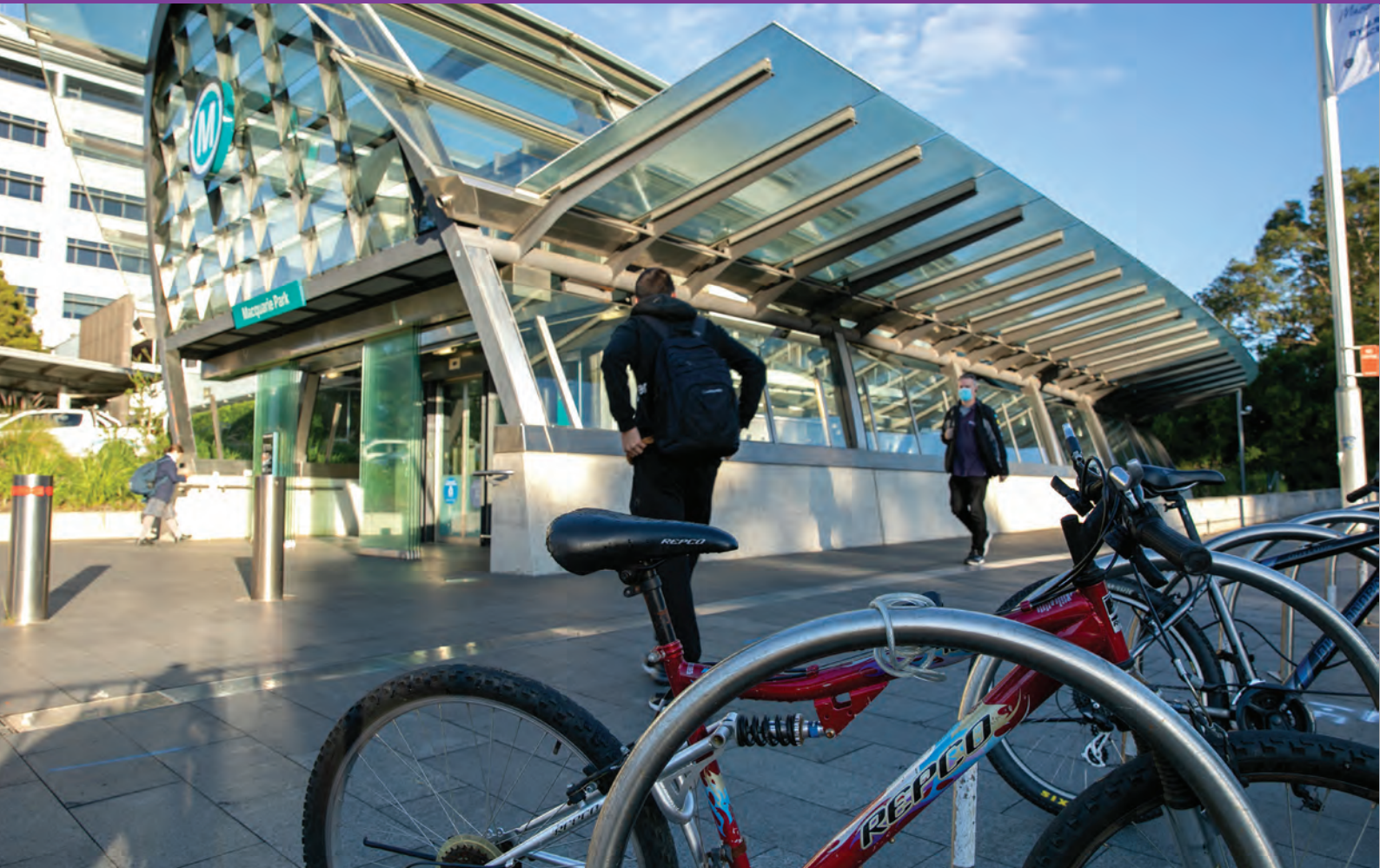
Bike racks, Macquarie Park train station.
