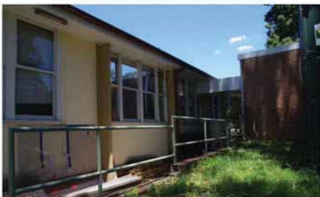
The north western side with the later addition for the upgraded extraction system.
