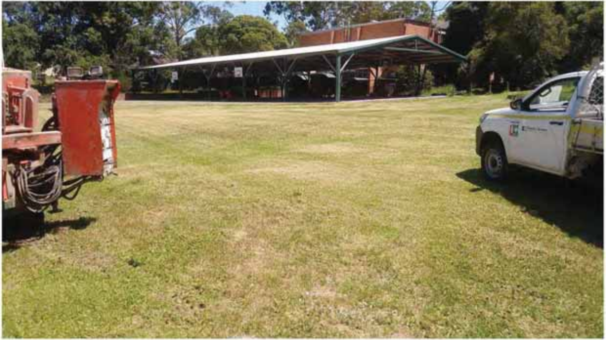
Photo 3: Drilling works in sports field.
