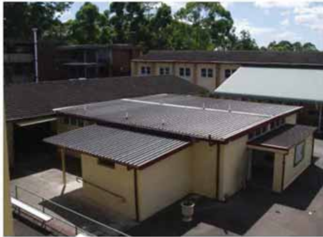
Building B00I as seen from Building B00A. Note the extension to the side. The entrance to the girls toilet is through the door to the right, with the boys toilet entrance on the opposite side.
