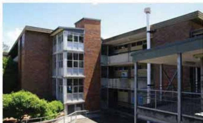
Building B00K (left), B00J (right) with the lift and stairwell between.
