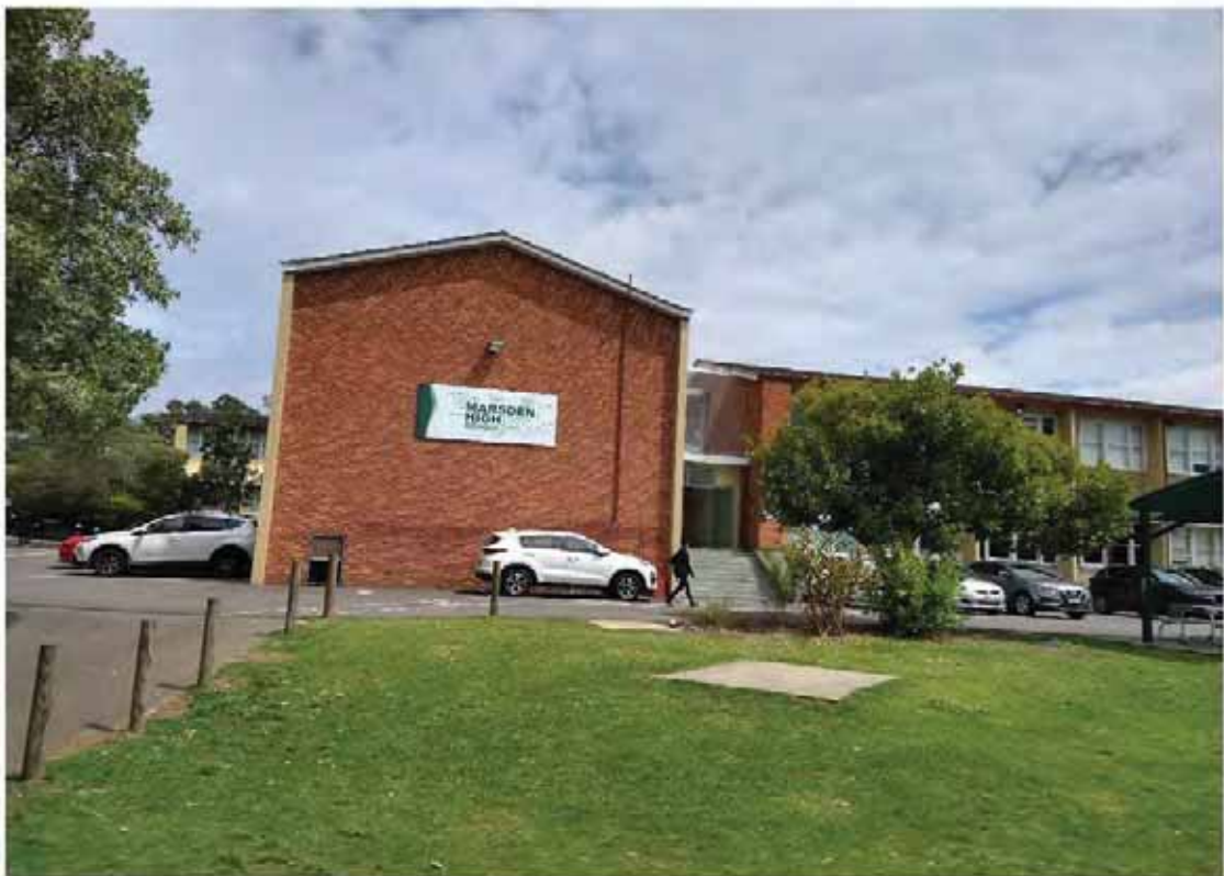
Photo 2: School building that back onto playing fields, north
