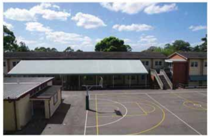
Building B00E (left and to the rear) and the link with B00D, viewed from B00A. Building B00I (formerly G) to the left.
