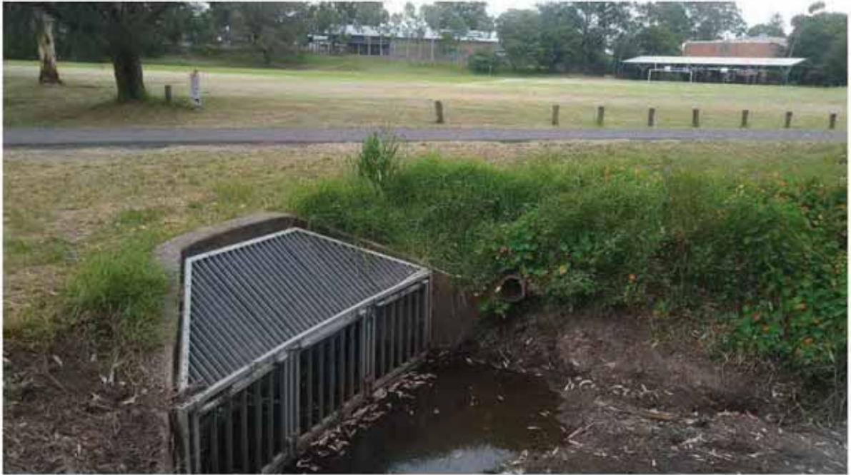
Photo 7: Archers Creek as it flows into the channel beneath the south eastern portion of site.
