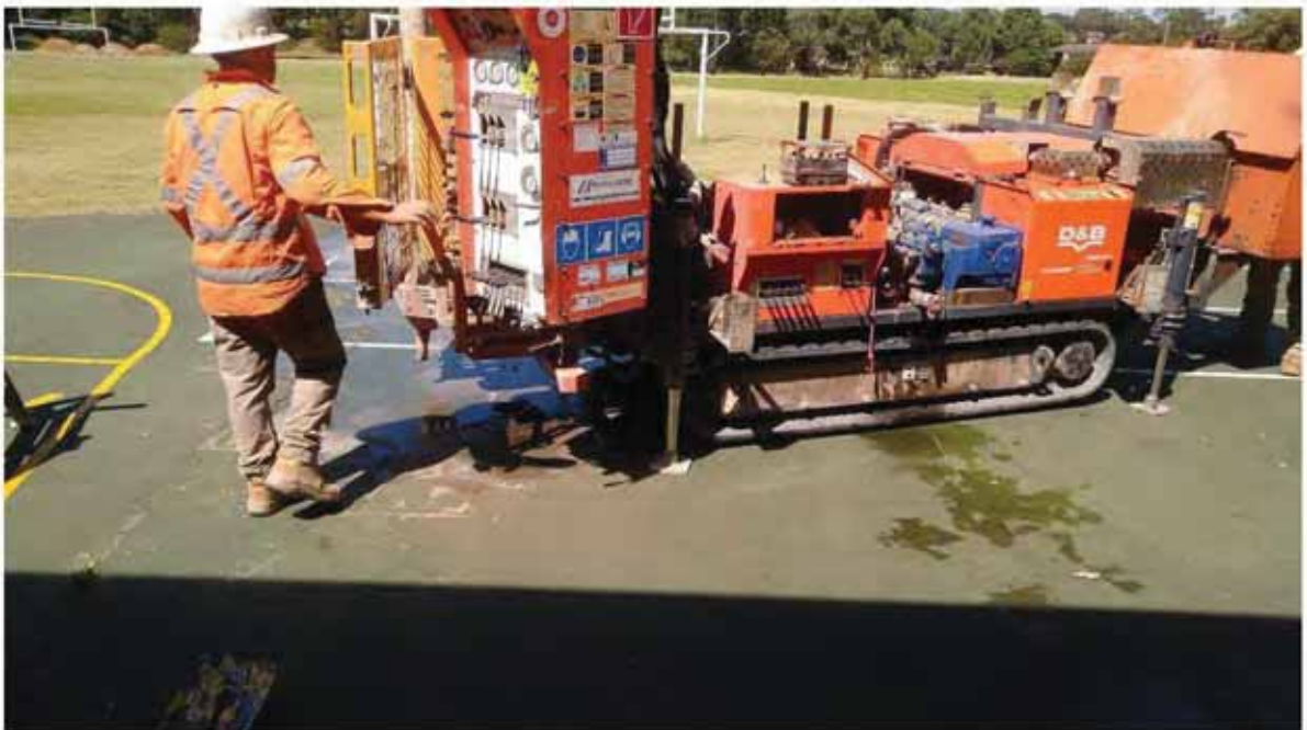
Photo 4: Drilling works in the hardstand playing court.
