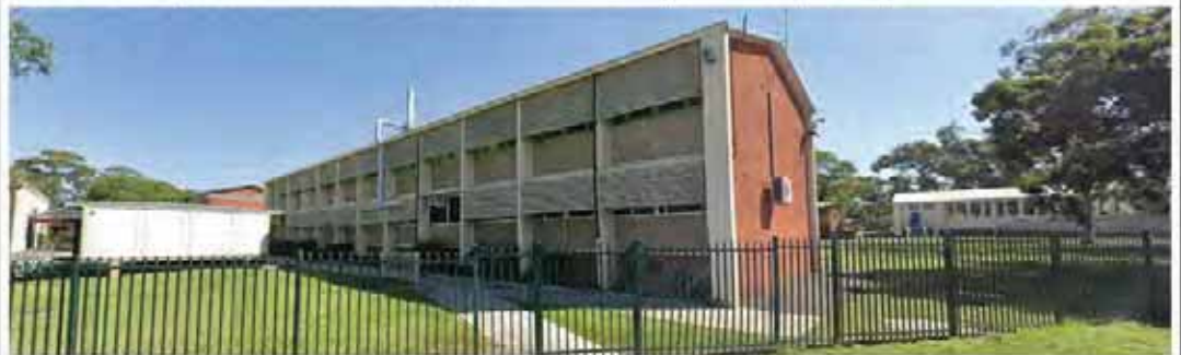
The roof material was unable to be ascertained from Google Street View, although the green colour of the roof on plan view is suggestive of its replacement with a coloured, profiled sheet metal roof. (Source: Google Street View October 2020)
