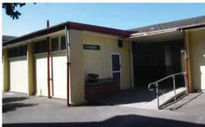
Tilt-up metal clad doors provide entrance to the shelter area.
