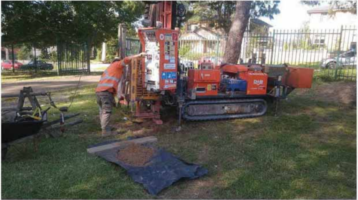
Photo 1: Drilling works in the north western portion of site.
