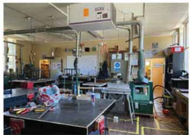
Wood Tech Learning space interior with upgraded extraction systems. The staff area is beyond the far door.
