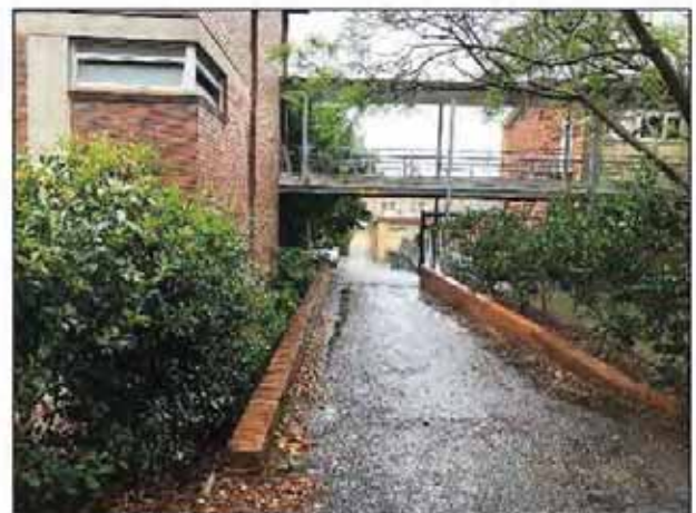
Photograph 4: View north west into school buildings
