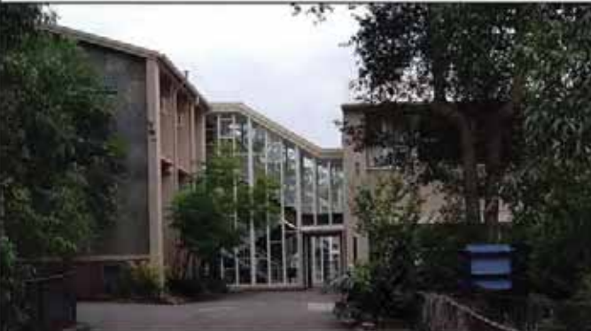
Typical classroom block connection, note exposed aggregate gable end. (Source: Purcell)
