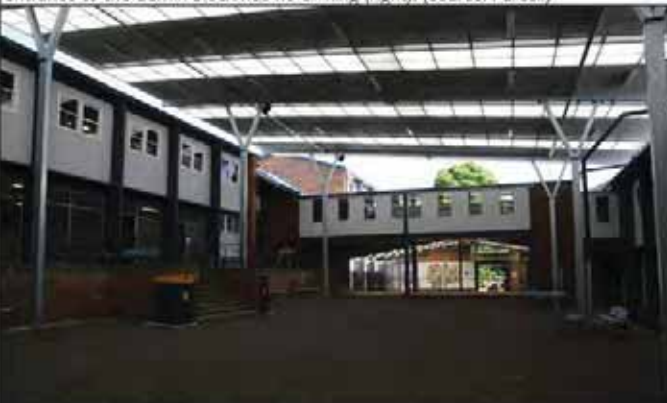
Canteen and shelter (left) with later COLA over the north east courtyard The link has been recently re-clad with profiled sheet metal. (Source: Purcell)
