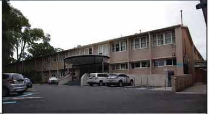
Administration block with semicircular awning (Source: Purcell)
