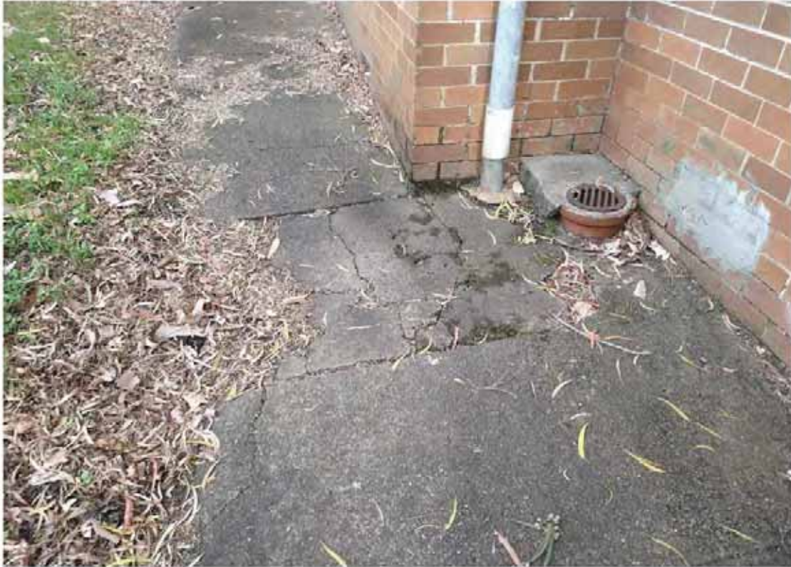
Photo 17: - Cracked concrete pavement similarly observed across the site
