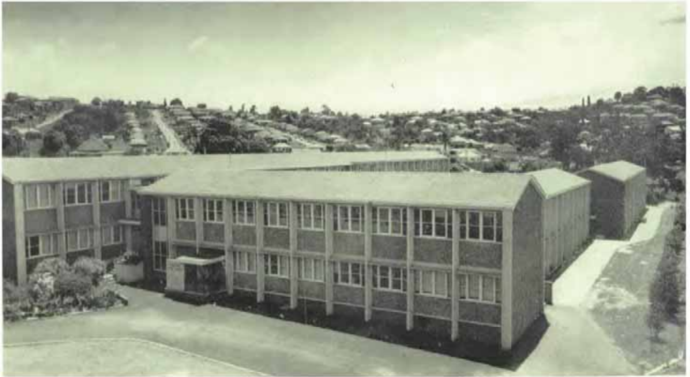
Marsden High School in 1965, the main entrance to Building B00C, Building B00B (left), and a view of Buildings B00D, B00E, and B00A behind (Source: SINSW)
