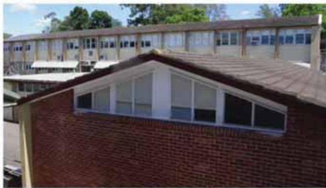
The gable end windows provide light into the covered shelter.
