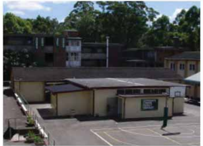
View of Building B00I from the top level of Building B00C. The tiled and metal roof sections can be seen in this image.
