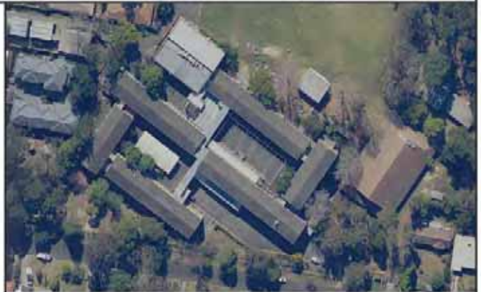
The north west building appears to be a 'Plan A library / laboratory block' 28 (1975) and north east building is the Hall (1984). (Source: SIXMaps, 2018)
