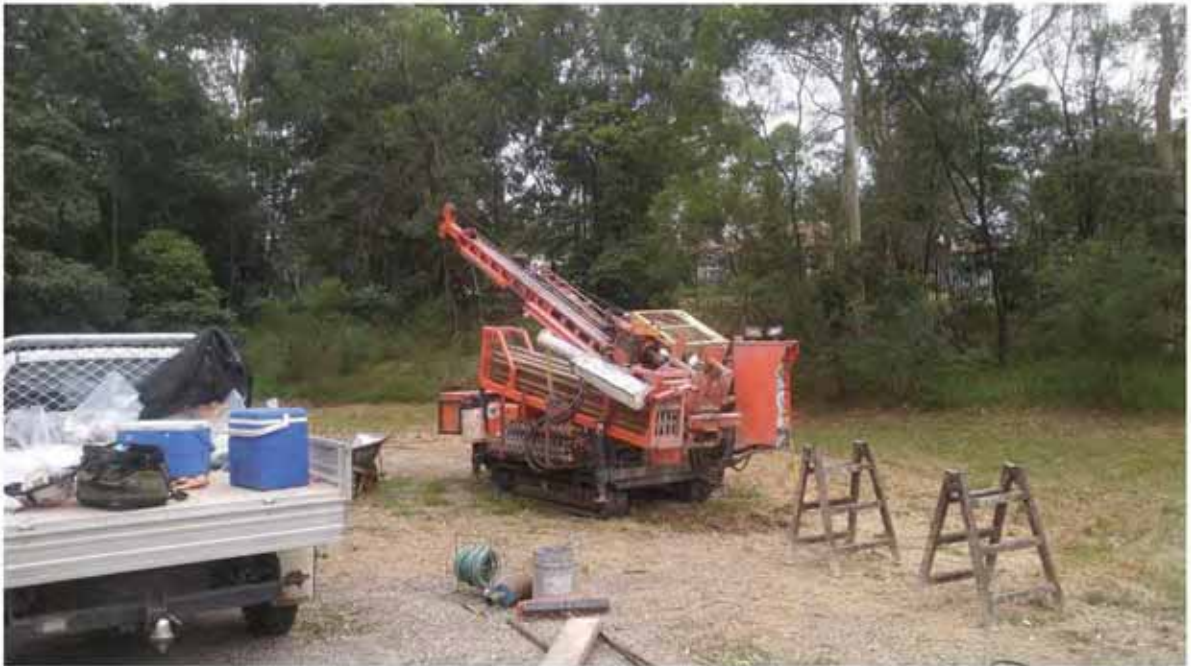
Photo 6: Drilling works in the eastern portion of site.
