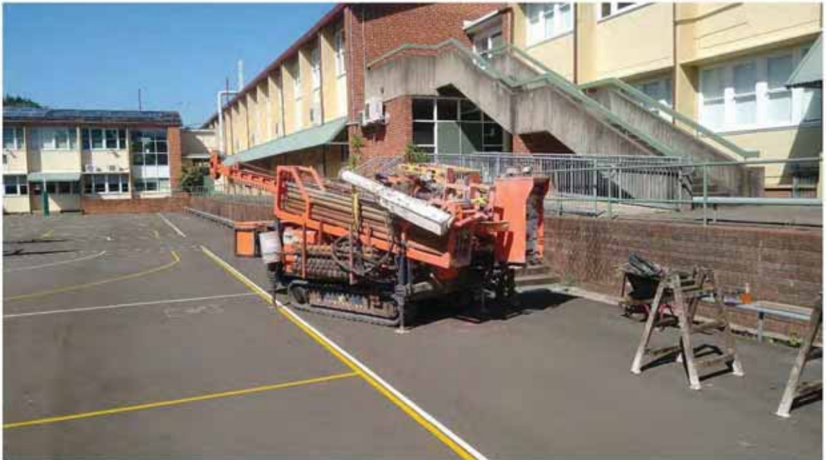
Photo 2: Drilling works within Marsden High School Courtyard.
