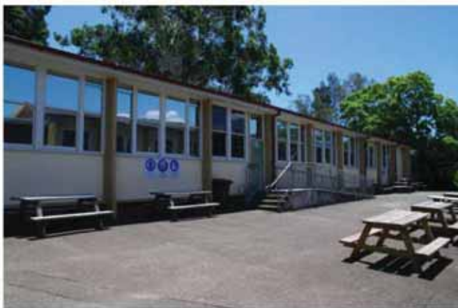
The middle of Building B00F with the later ramp and stairs added for accessibility.
