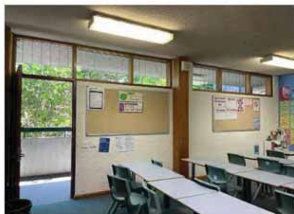
Typical classroom in Building B00J note the timber framed louvre windows to the external corridor with off-form concrete balustrades.
