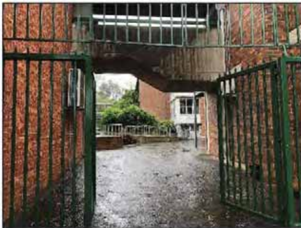
Photograph 1: View north west into school buildings
