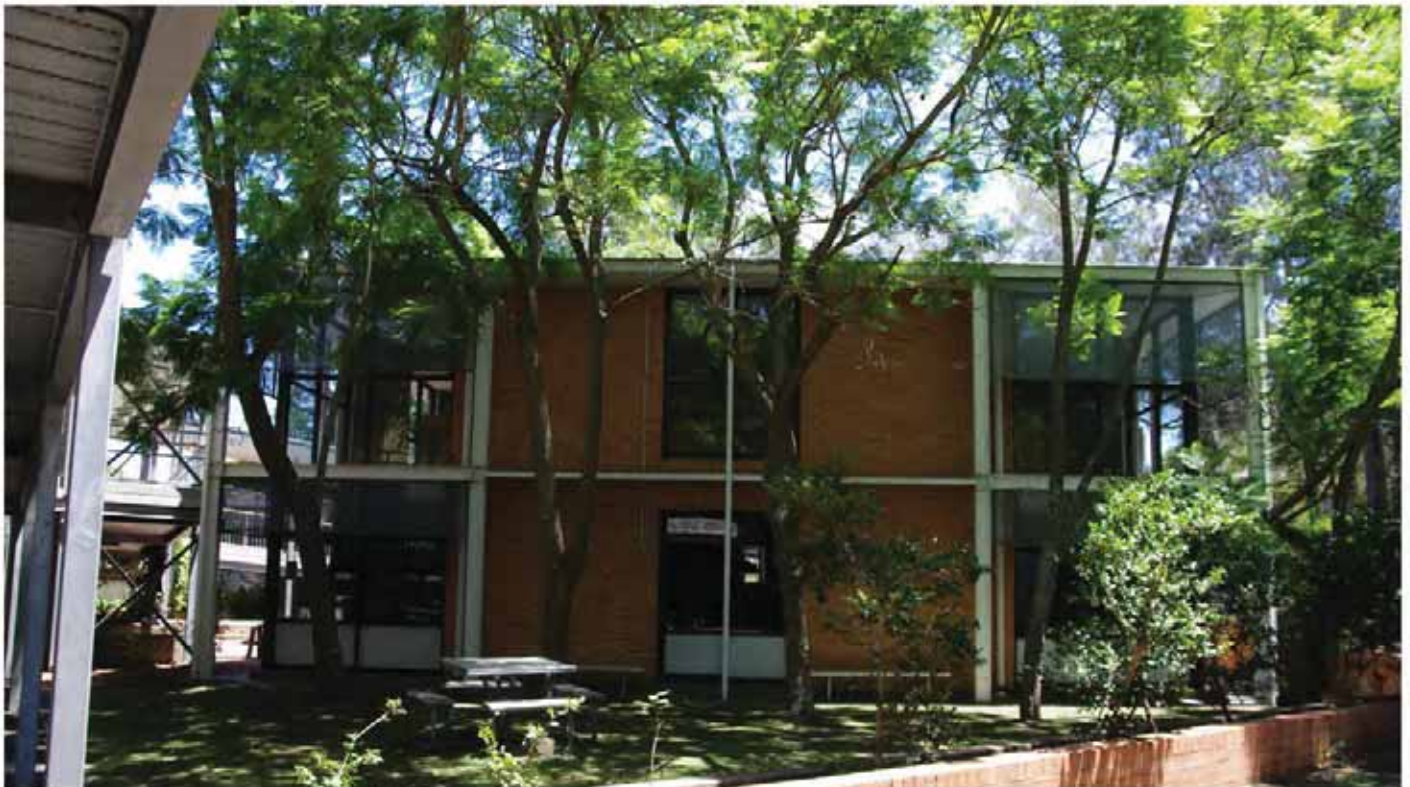
The Library (Building B00G) with the covered walkways connecting it to Buildings B00A and B00K
