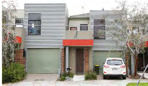
Example of contemporary 2 storey front loaded terrace houses (Source: Moreland City Council)
