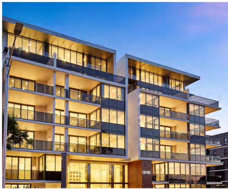
Modern mid-rise apartments
