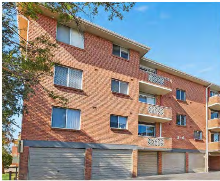
Older low-rise apartments
