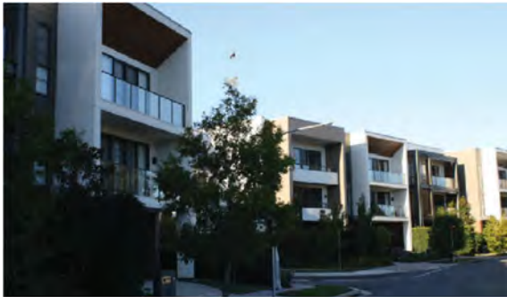
Putney Hill's terrace houses are a good example of a 3 storey typology providing surveillance to the street
