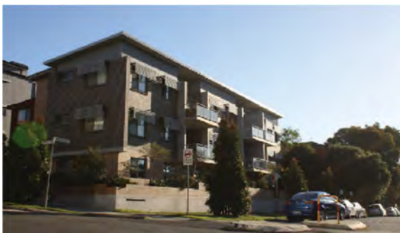
A more traditional (older) 3 storey low rise apartment building in Top Ryde is a frequent typology across Sydney
