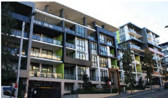
This medium rise apartment typology in Meadowbank is located along a steep frontage
