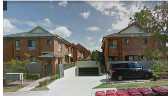
A townhouse development in Ryde with basement parking located in an R3 zone
