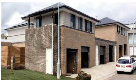
Example of an affordable 'fonzie flat' in the Potts Hill Community Housing precinct in Bankstown
