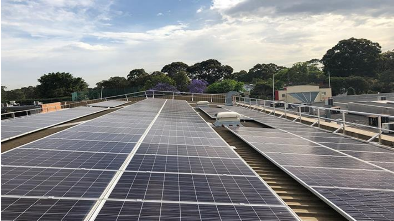
Solar panels at the North Ryde School of Arts Community Centre
