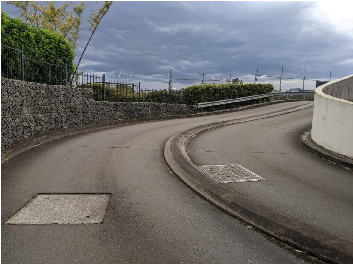
Figure 5: Internal Access Ramp from Ground Level Carpark to Basement Carpark (Humceptor lid at left of image)
