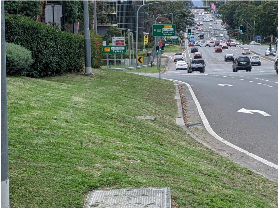
Figure 2: Batter from site to Lane Cove Road and series of road kerb inlet pits
