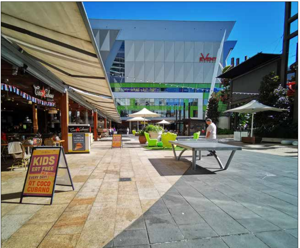
Public plaza in Top Ryde delivered through redevelopment
