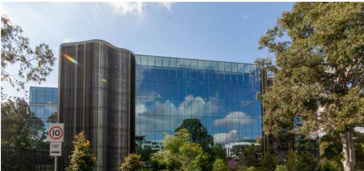
Novartis Building Waterloo Road, Macquarie Park
