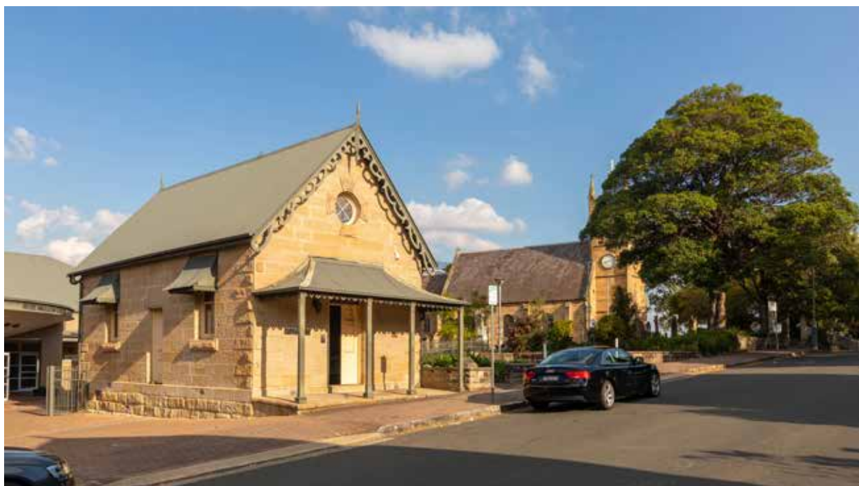
Church Street heritage precinct, Ryde
