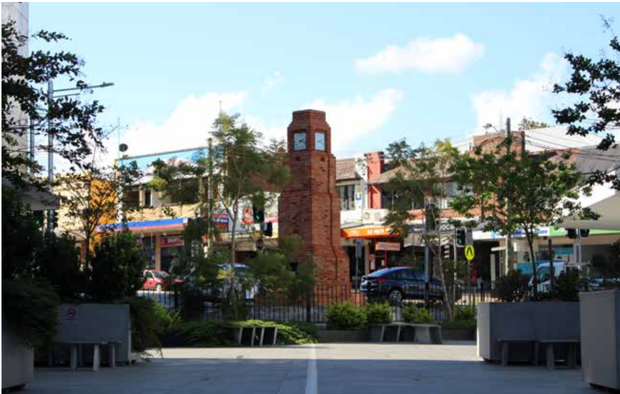
Recently restored the Sheridan Memorial Clock, Gladesville
