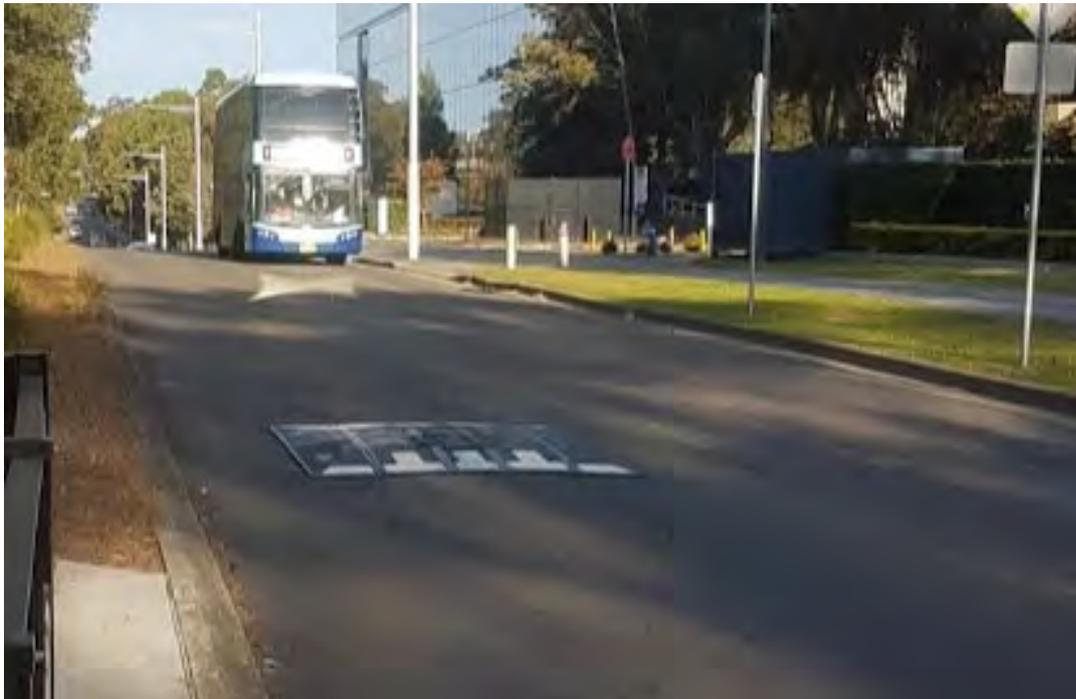
Figure 21 Recommended speed hump types
