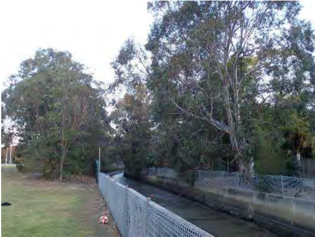
Figure 94 Revegetation areas line the banks of channelled creeks where they pass through Meadowbank Park
