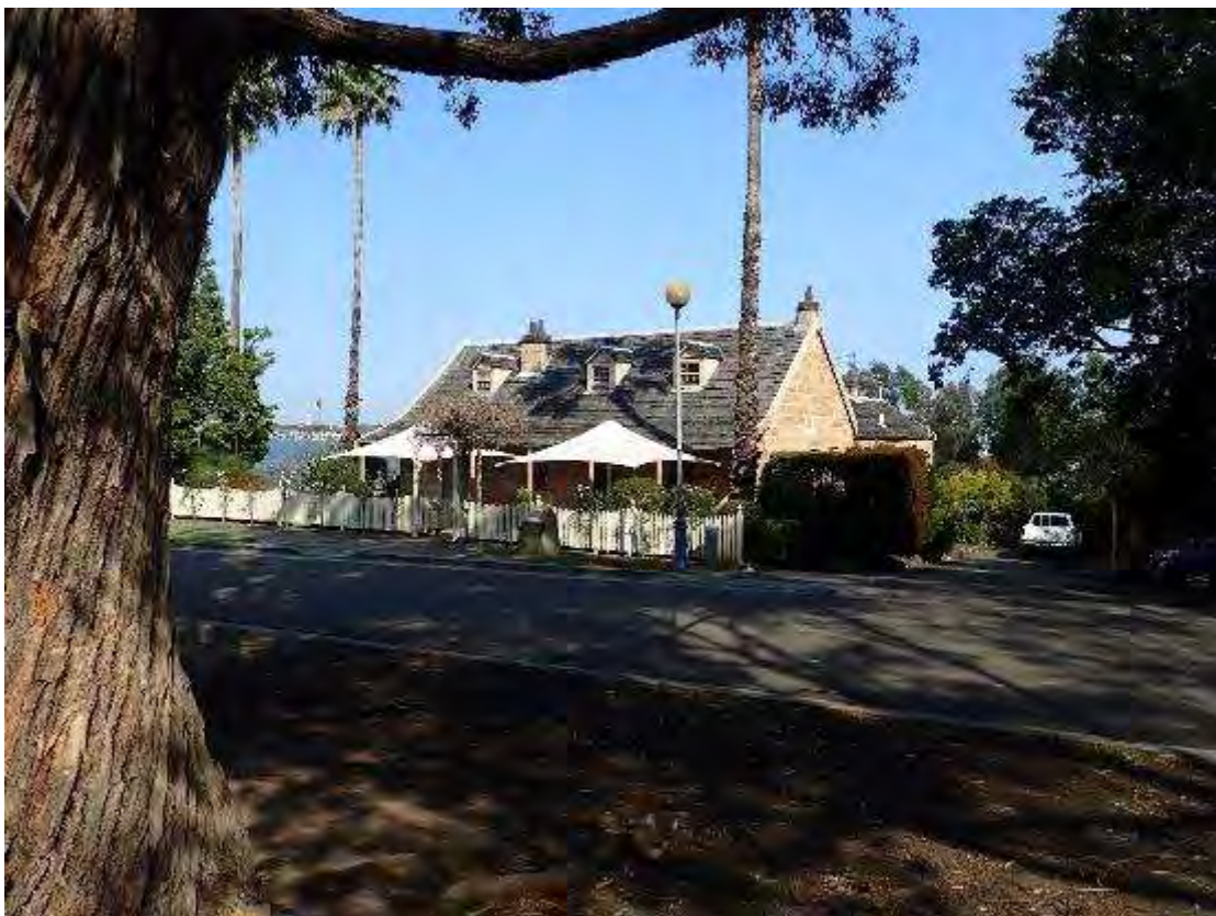
Figure 22 Banjo Patterson's house is a central point to this reserve
