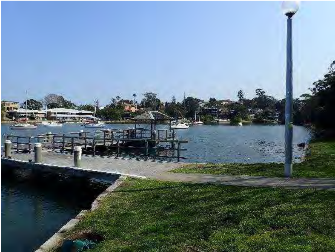
Figure 21 Much of the foreshore area is managed lawn behind retaining walls, especially near the wharf
