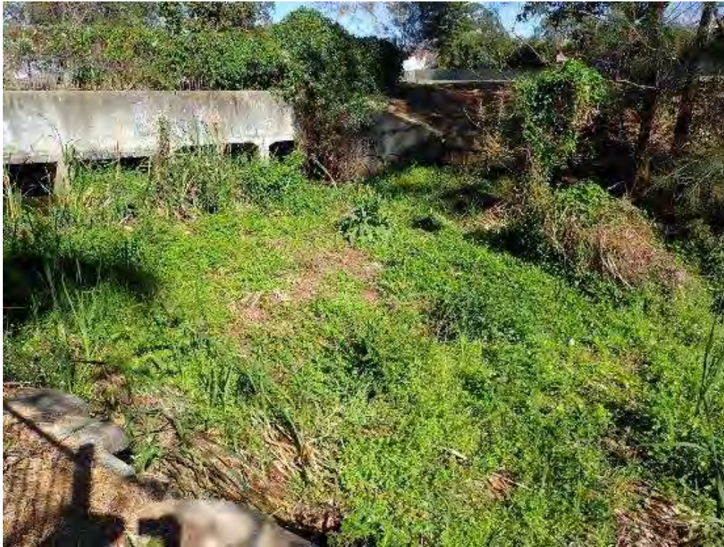
Figure 181 Dense weeds fill the channel where Shrimptons Creek daylights into Santa Rosa Park
