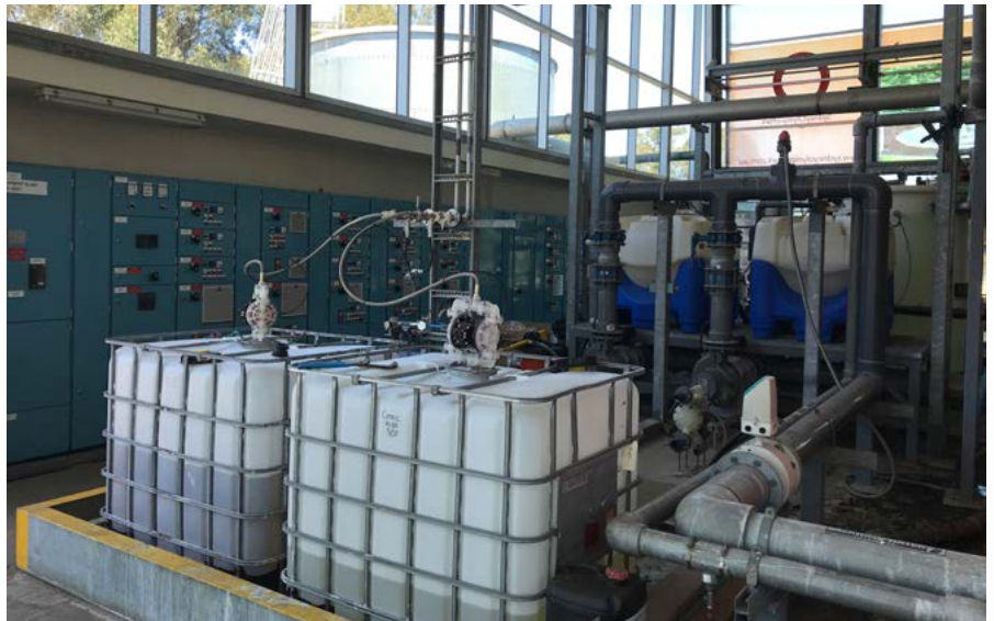
Pictured: Water recycling facility
