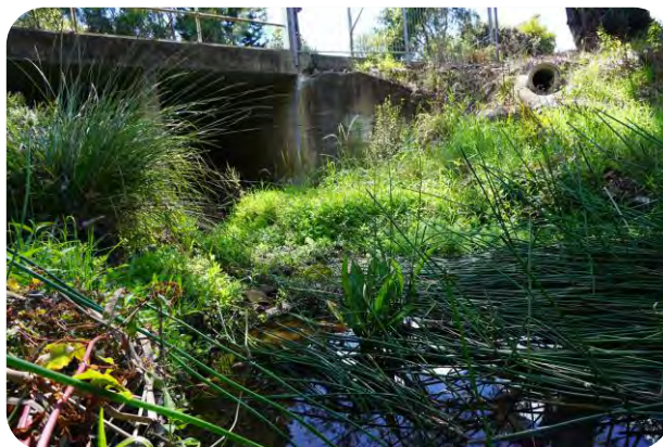
Figure 13 Shrimptons Creek @ Bridge Street facing downstream
