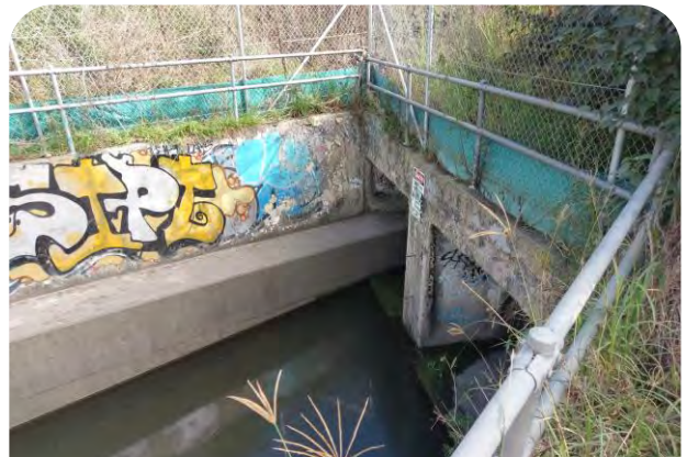
Figure 34 Porters Creek @ Main Branch facing downstream
