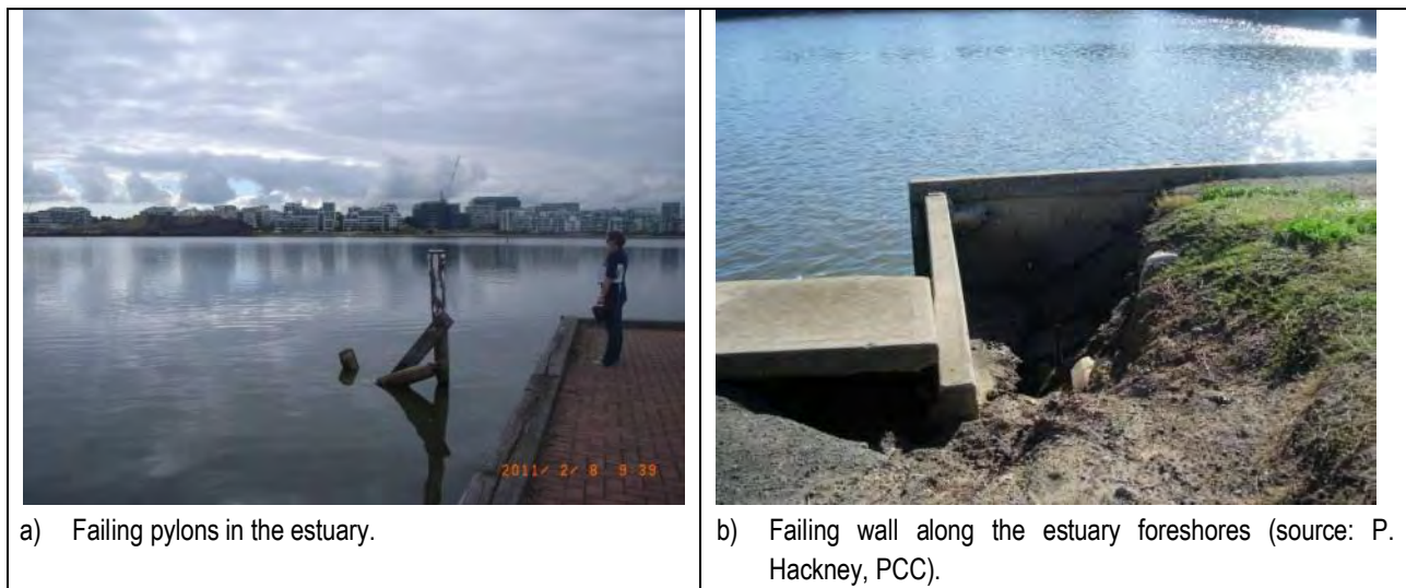
Figure 2.30: Failing Foreshore Infrastructure
