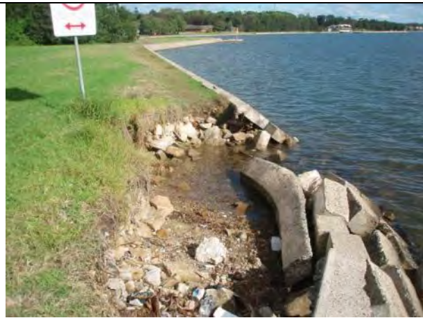
Failed seawall, Leichardt (source: D. Wiecek, OEH, date unknown).
