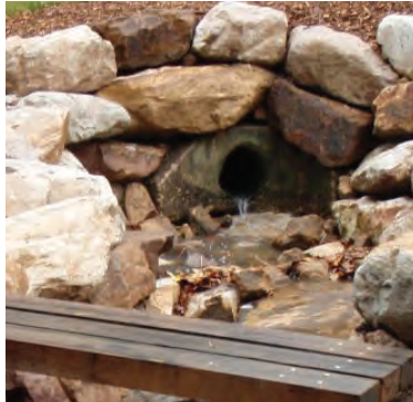
Rock lined headwalls and drainage lines to stormwater water outlets to manage erosion, before flowing to planted bio swales.
