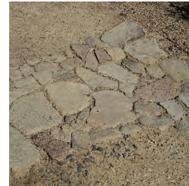
Track features - stormwater management using a stone lined invert.
