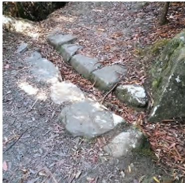
Track features - stormwater management using a stone gutter / box drain.
