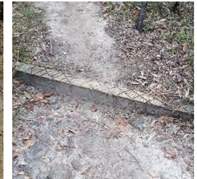
Track features - stormwater management using a sleeper water bar.
