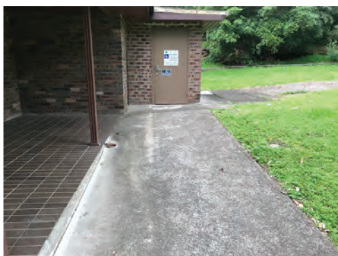
The accessible toilet on the southwest side of the Visitors Centre / Amenities Building is separated from the internal access way by a grassed area (access does not comply with accessible requirements).
