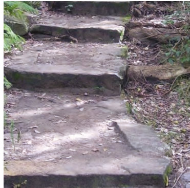
Track features - stone step and runs with compacted fill treads.
