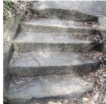
Track features - steps cut into insitu rock.
