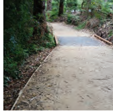
Accessible park path of crushed sandstone or compacted gravel with timber edge boards.
