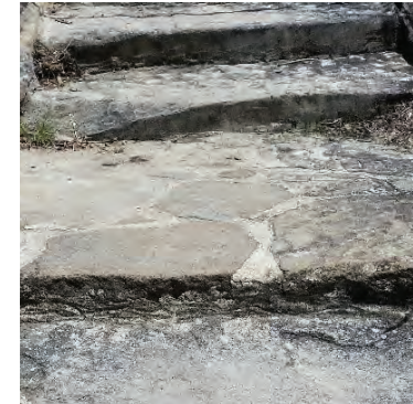
Track features - infill stone flagging and rock leveling to create a passable track over insitu rock outcrops.
