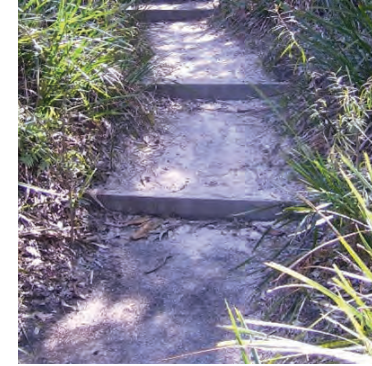
Track features - sleeper step and runs with sand or compacted fill treads.
