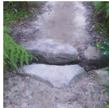
Track features - rock lined box drain / gutter.
