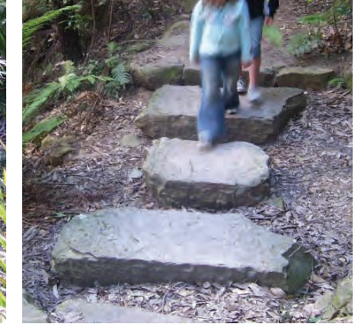
Track features - stepping stone creek crossing.
