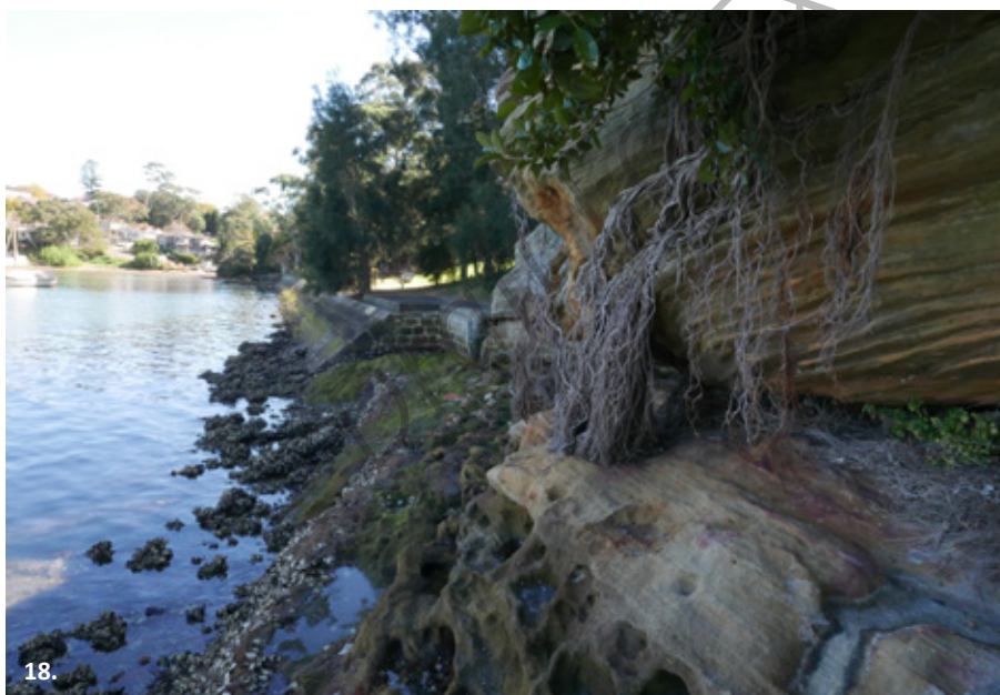
18. The seawall at Banjo Paterson Park is in poor condition. There is opportunity to provide continuous foreshore access as part of the upgrade to the seawall edge.
