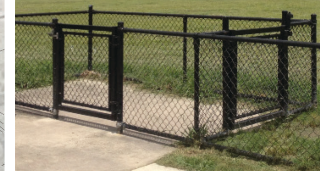
ENTRY/ EXIT AIR LOCK GATE AND CHAIN LINK WIRE FENCE
