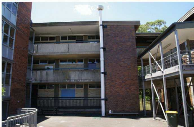
Building B00J (centre), link between Building B00H (right).
