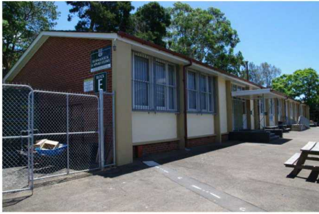
The south elevation of Building B00F with the main entrance under the portico.
