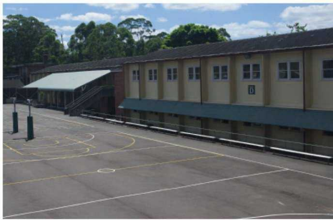
Buildings B00E (left) and B00D (right) note the difference in fenestration compared to Buildings B00A, B00B, and B00C.
