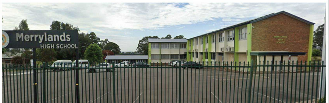
The roof has been replaced with profiled metal sheeting since 2018. (Source: Google Street View, October 2020)
