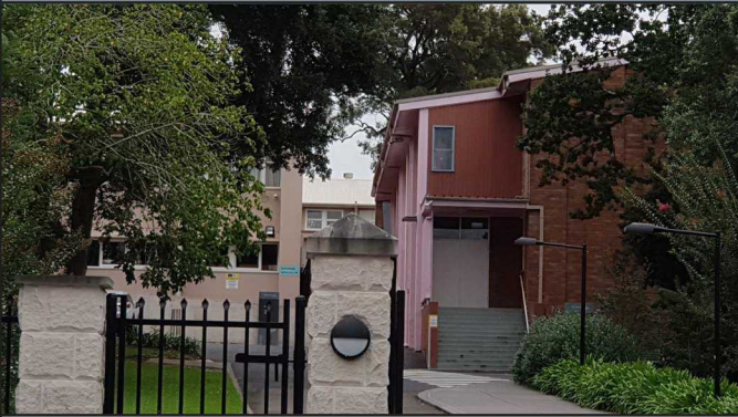
Front entrance with contemporaneous Hall (right). (Source: Purcell)
