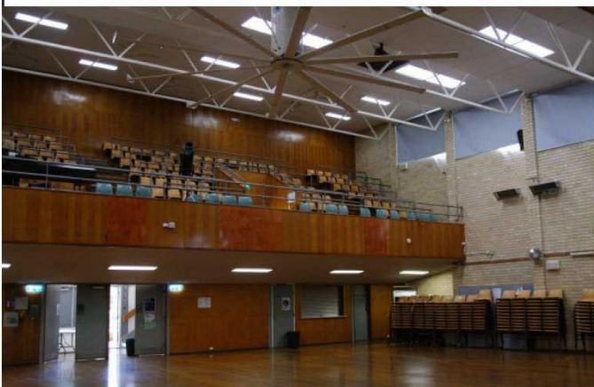
The mezzanine above the front entrance. Note how the ceiling steps down towards the stage.
