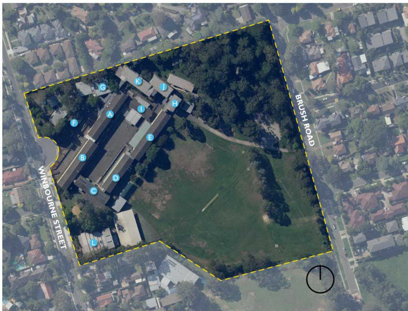
Marsden High School Buildings, future boundary shown dashed in yellow (Source: SIXMaps modified by Purcell, boundary information supplied by SINSW)
