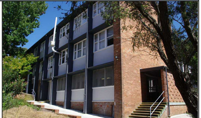
The sloping block was utilised to create a third level for a change room. The fenestration is similar to Marsden HS. (Source: Purcell)
