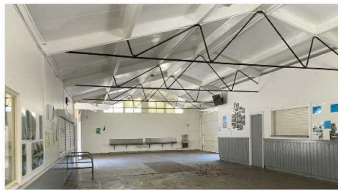
The interior of the covered shelter area, with the Cafeteria to the right.
