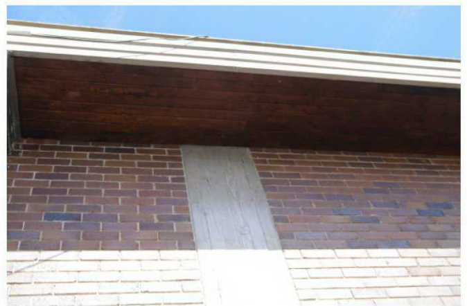
Detail of the timber eaves to Building H.
