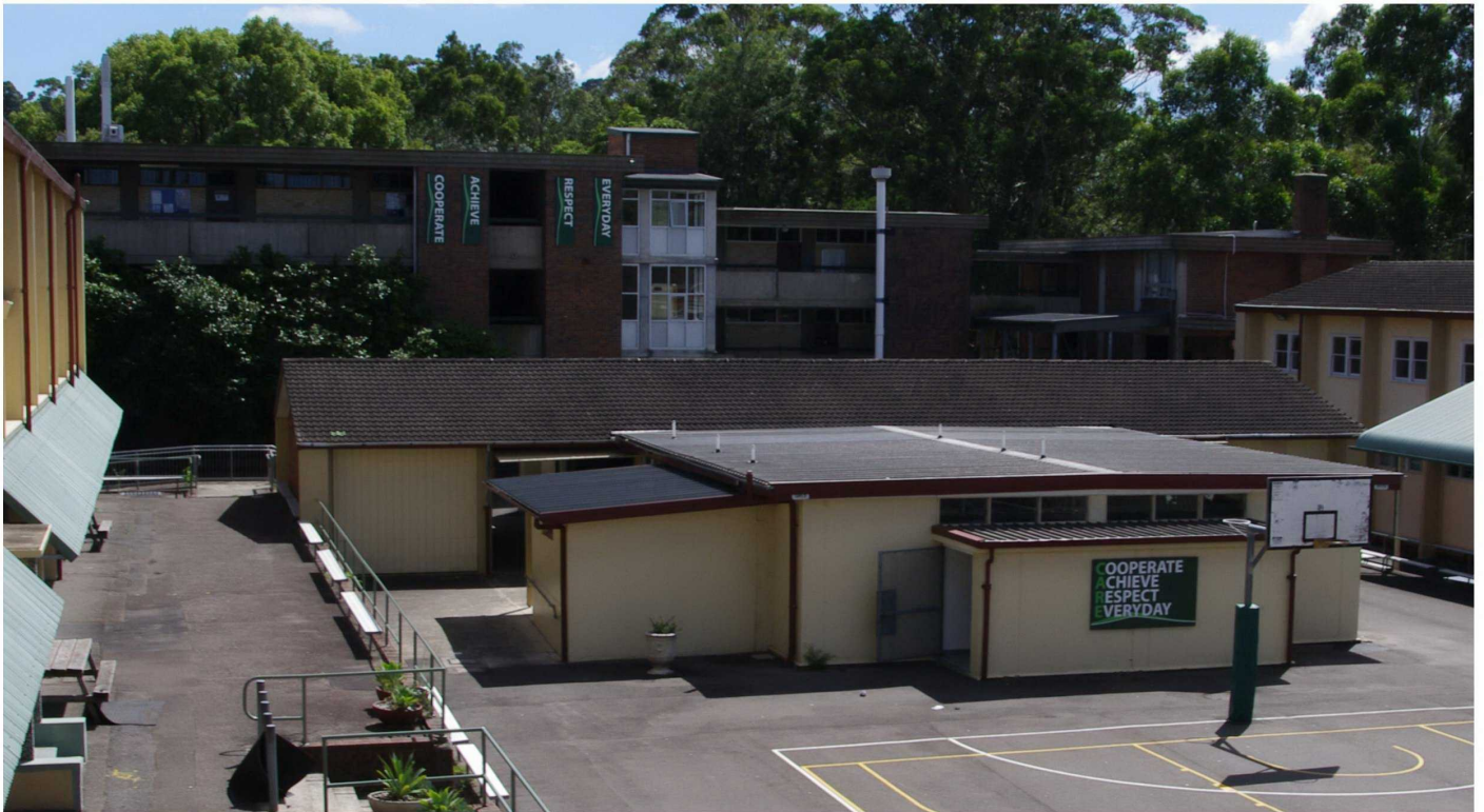
Pupil Facilities and Food Services Unit (Building B00I - formerly G, Stage 1) with the 1971 additions behind: Buildings B00H - right, B00J - centre and B00K - left
