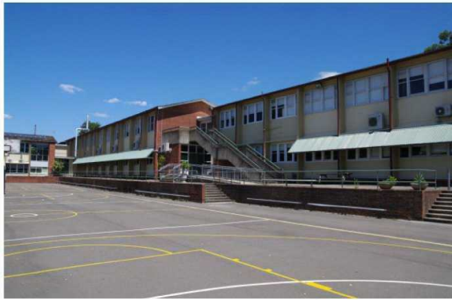
Buildings B00A (right), B00B and B00C (left) from the Sports Court.
