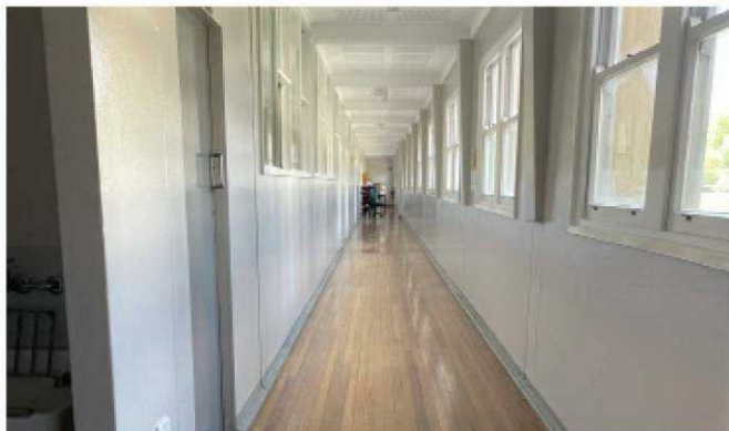
Typical single-loaded corridor layout with potentially original timber floorboards.
