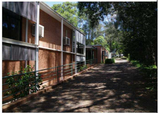
Current view of the north west elevation. The building is obscured by the ramps, covered walkway and landscaping.
