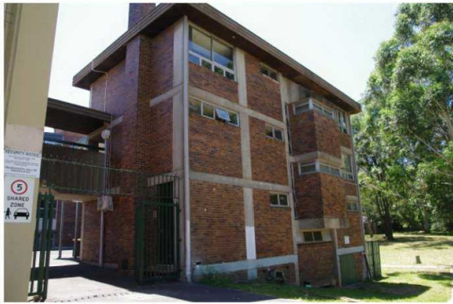
Current view of the north east elevation of Building B00H. Note the exposed off-form concrete.
