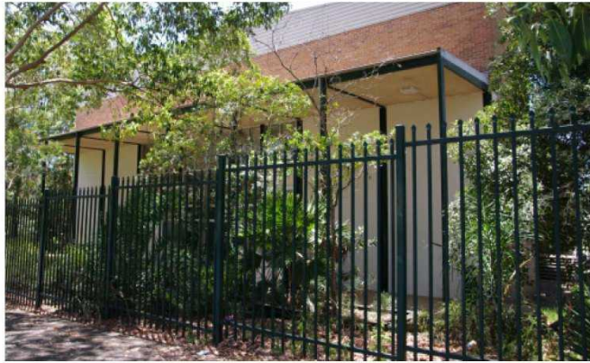
The Winbourne Street elevation is the main entrance to Building B00L and is obscured by landscape planting.
