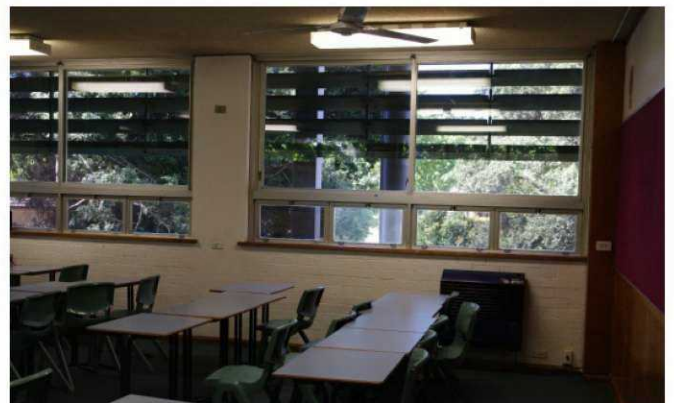
Building B00K has exterior louvred window sunshades (as seen from inside a classroom).
