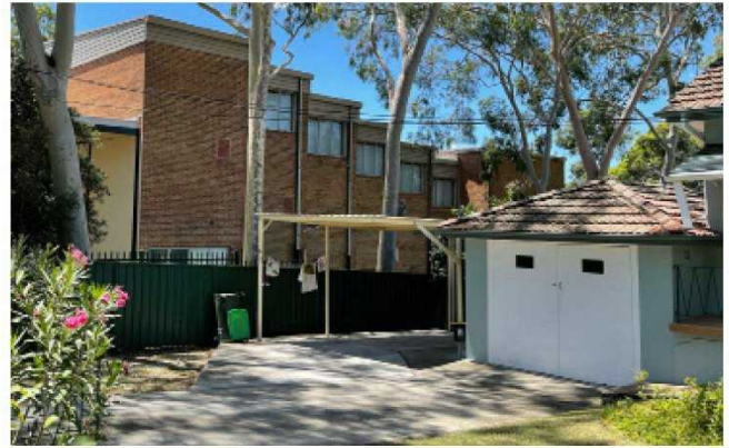
Current view of the southern side of the building showing the stepped walls and roof. The building is obscured by landscaping and the adjacent residential houses.
