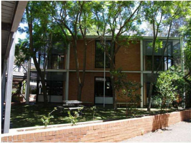
The north side of Building B00G, showing the face brick walls and corner glazing.
