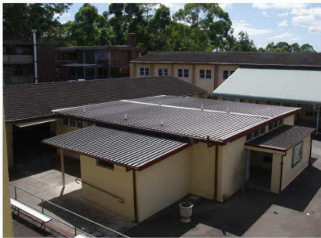
Building B001 as seen from Building B00A. Note the extension to the side. The entrance to the girls toilet is through the door to the right, with the boys toilet entrance on the opposite side.
