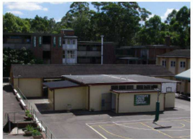
View of Building B001 from the top level of Building B00C. The tiled and metal roof sections can be seen in this image.
