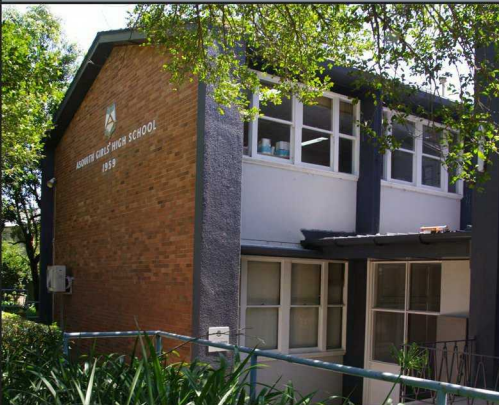
School signage is installed on the gable end, similar to Marsden HS. Note the entrance to the admin block has no awning (right). (Source: Purcell)
