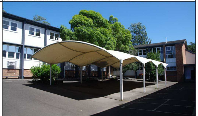
The north west courtyard with COLA. All standard fenestration patterns are shown, stairwell (right), large and small (left). (Source: Purcell)
