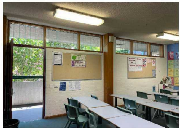
Typical classroom in Building B00J note the timber framed louvre windows to the external corridor with off-form concrete balustrades.
