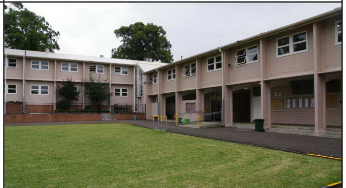
Typical classroom blocks looking north west across the courtyard. Note the original tiled roof was recently replaced with a sheet metal roof. (Source: Purcell)
