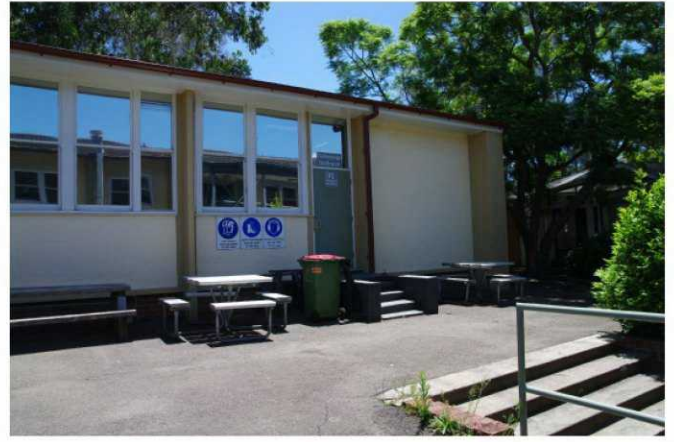
Current view of Building B00F. Note the end bay without windows where the staff toilets are.
