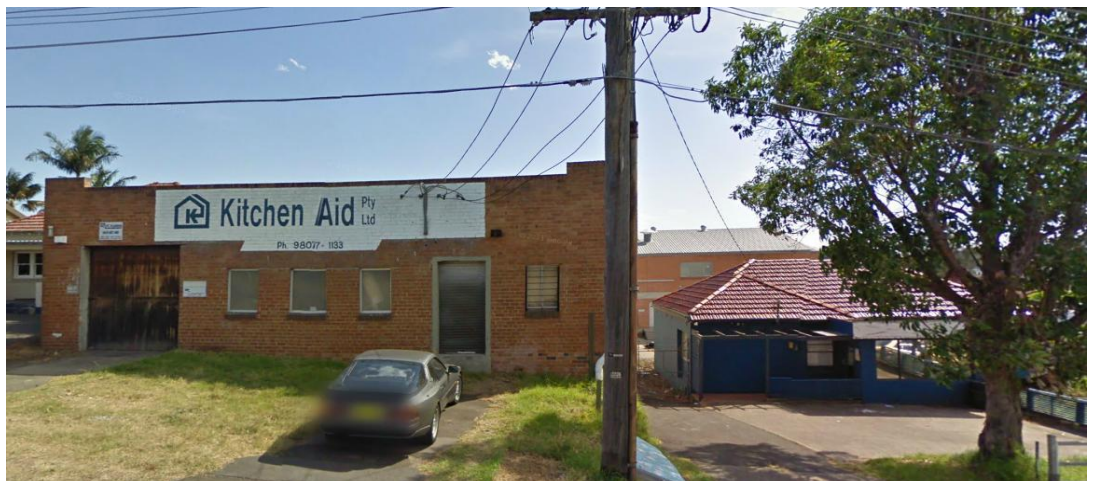
Figure 8: Existing Development South from Nancarrow Avenue (Source: Google Maps, 2009)
