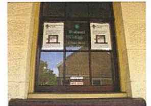
Figure 26b: Original Front Window
