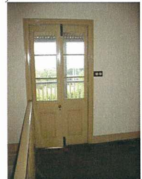
49b Ground Floor – French doors to Westward Cottage's Balcony
