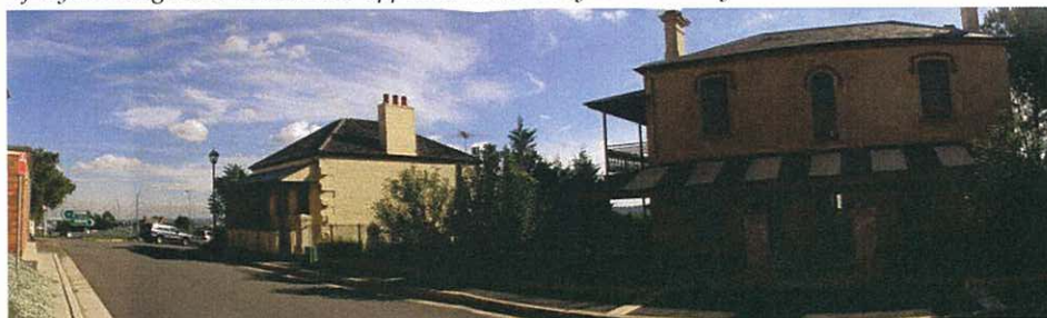
Figure 28: View from the corner of Turner Street of the streetscape setting of Westward Cottage. The Parsonage, a former Wesleyan Ministers Residence is situated in the foreground to the south of the cottage.
