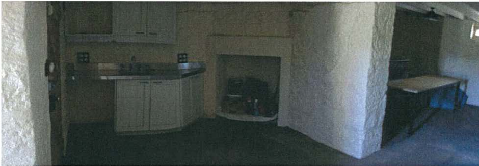
Figure 48: Rough rendered reconstructed stone walls to Lower Ground Floor. Fireplace represents an open Colonial Kitchen Fire.
