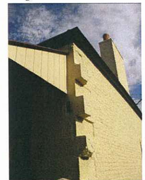
Figure 26c: The corner showing toothed sandstone faithfully reconstructed.
