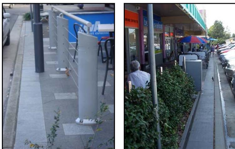
**Figure 4 Examples of suitable kerbside barriers**
