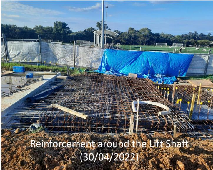
Reinforcement around the Lift Shaft
