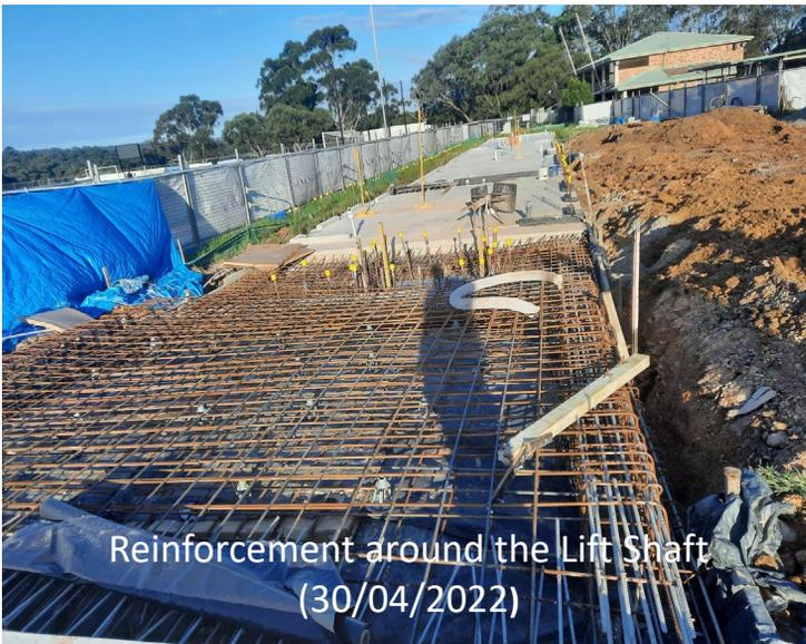
Reinforcement around the Lift Shaft
