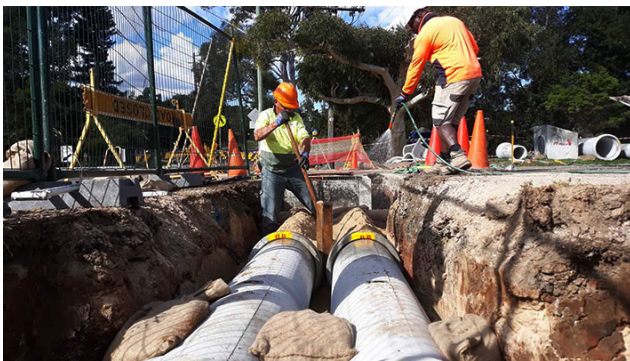
Example stormwater drainage works in progress
