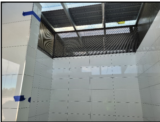
Wall Tiles Installation
