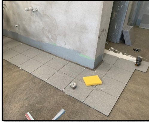
Floor Tiles Installation
