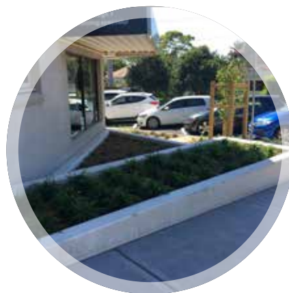
Avon Road construction complete
