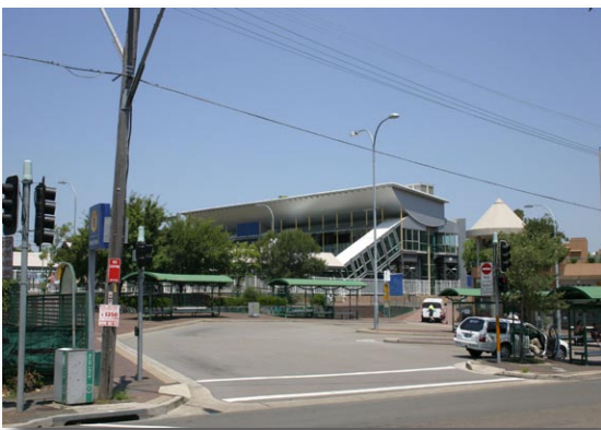
West Ryde Train Station
