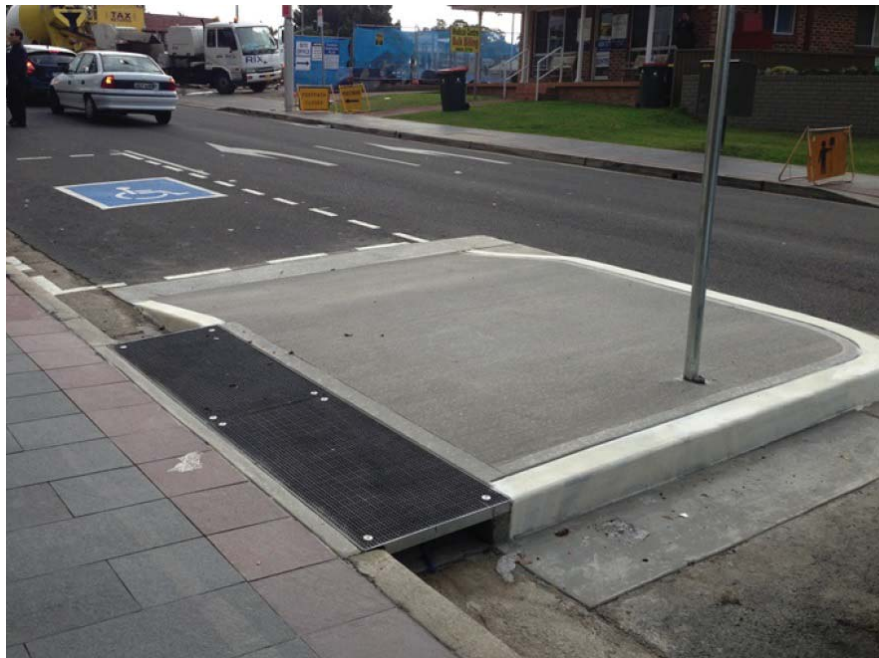
Part of the Footpath Renewal Program by Council to improve the taxi rank on Pope Street which services the Ryde City Shopping Centre.
