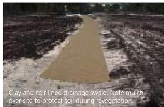
Clay and coir-lined drainage swale. Note mulch over site to protect soil during revegetation.
