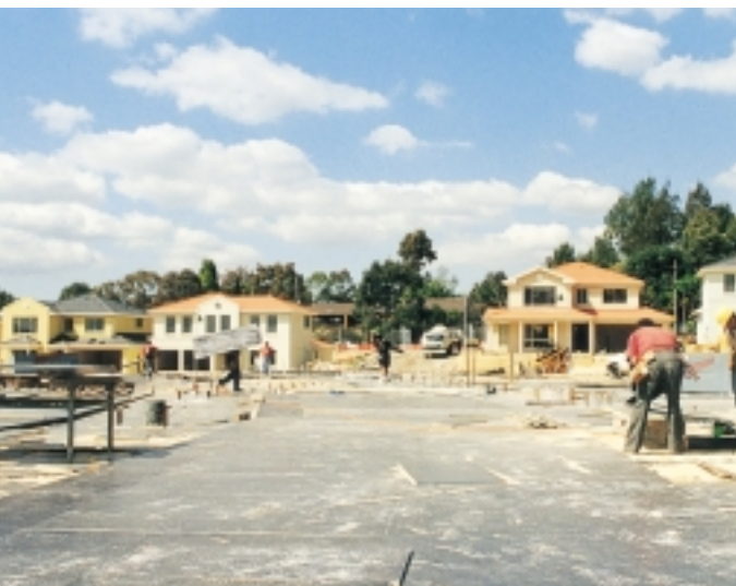
Construction well underway at Nile Close
