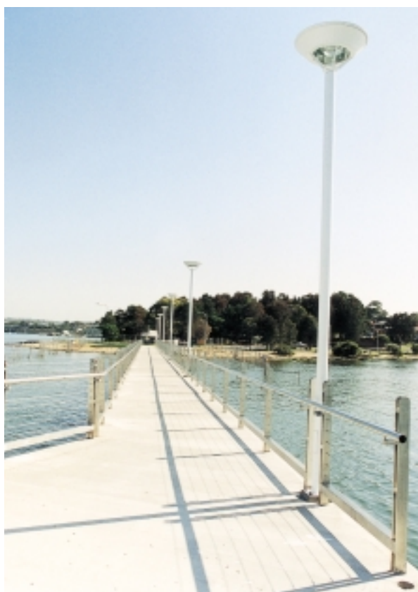
Kissing Point Wharf under construction
