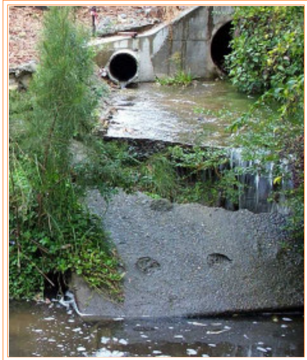
A major creek rehabilitation project on Archers Creek at Maze Park, West Ryde has commenced
