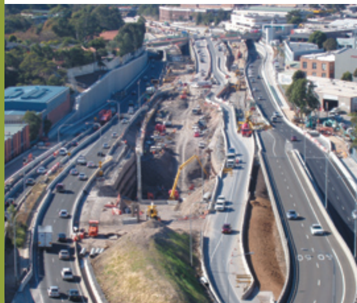
The Lane Cove Tunnel under construction
