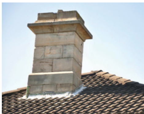
Detailed view of the sandstone chimney. Photo source: Ryde Library.
