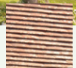
Terracotta shingle tiles roof cladding.
