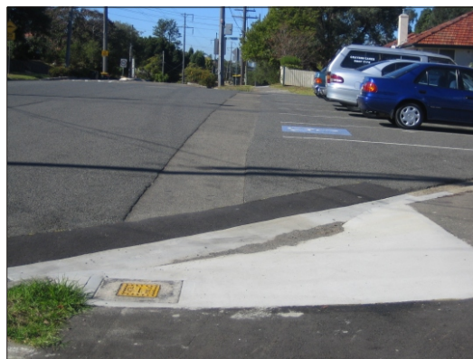
Drop kerb angled towards middle of road and not to the disabled parking space. No tactile paving used.
