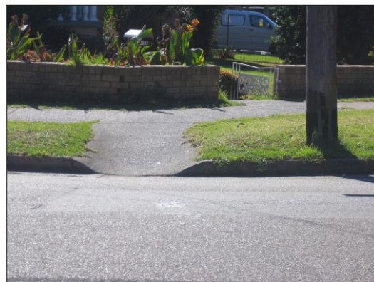
Steep and narrow drop kerb which does not line up with drop kerb on opposite side of road.
