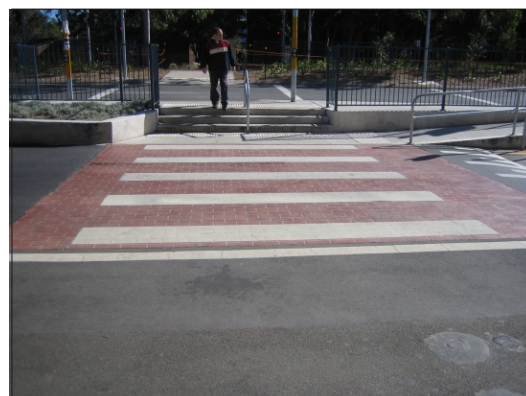
Dropped kerbs and tactile paving provided at signals but not at kebra crossing. Indirect route for mobility impaired and parents with prams.
