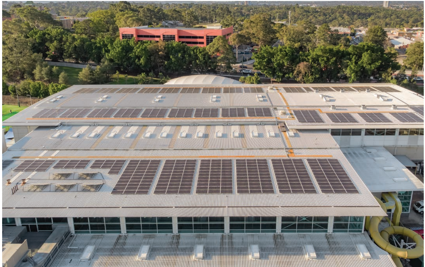
Photo: Ryde Aquatic Leisure Centre – Existing solar panels.
