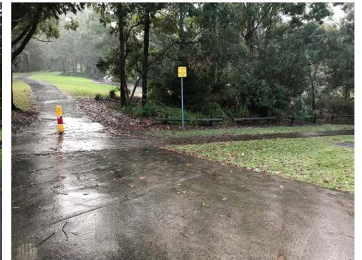
Drainage issues along Blenheim Road
