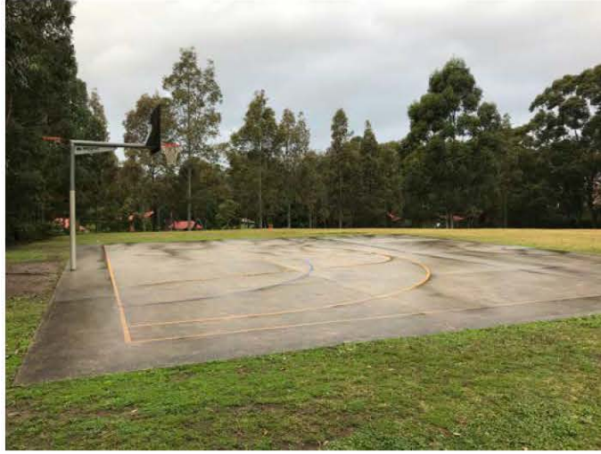
Existing Basketball half court with netball ring
