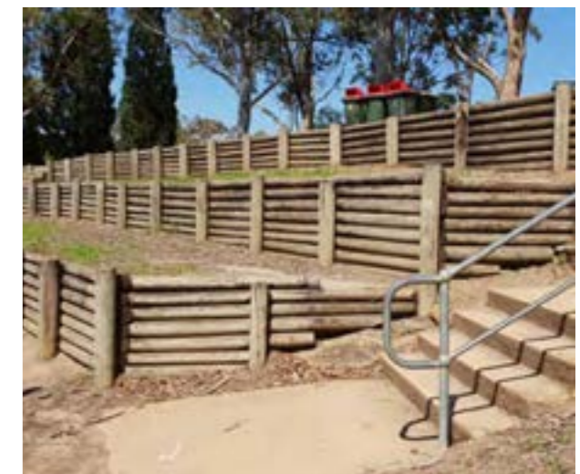
Ageing infrastructure adjacent to field 3
