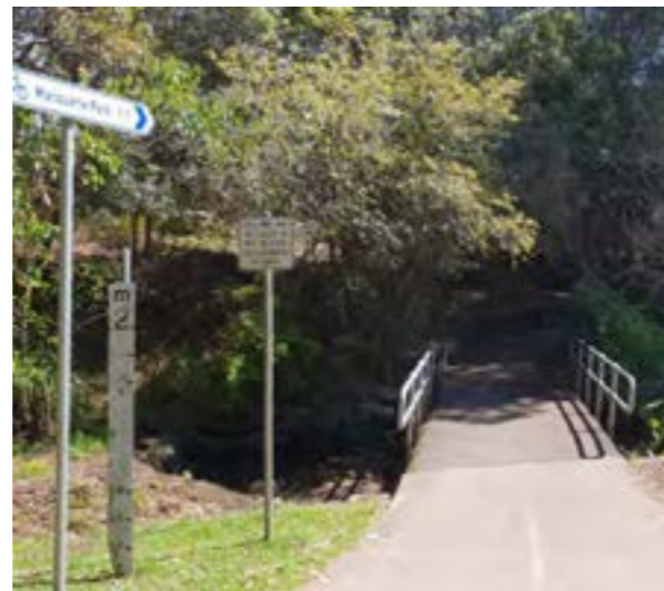
Shrimptons Creek shared path is well-used but flood prone
