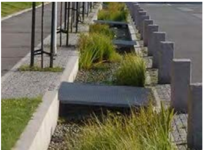
WSUD to car park
