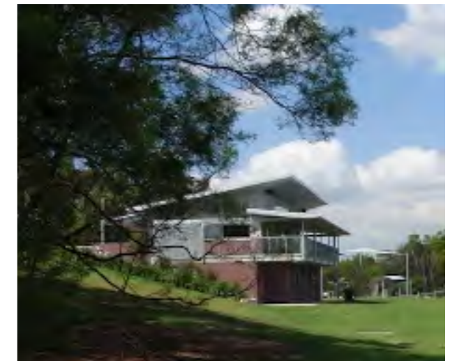
Seaforth Oval amenities - sporting amenities, canteen and store at field level with club rooms and viewing deck above
