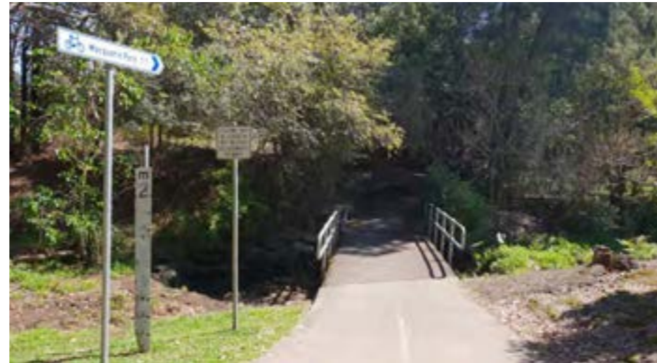
Existing Shrimptons Creek shared path and bridge crossing. Bridge proposed to be replaced and lifted to improve flood resilience. New lighting to be provided along pathway.
