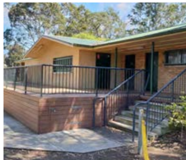
Former amenities building between fields 1 and 3. Building severely damaged by fire in February 2019.
