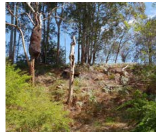
Bank erosion to Shrimptons Creek corridor
