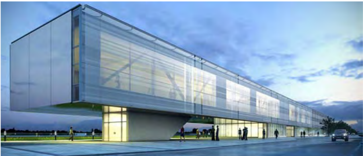
Laurier Brantford YMCA Athletics Complex by Cannon Design - elevated sports facility
