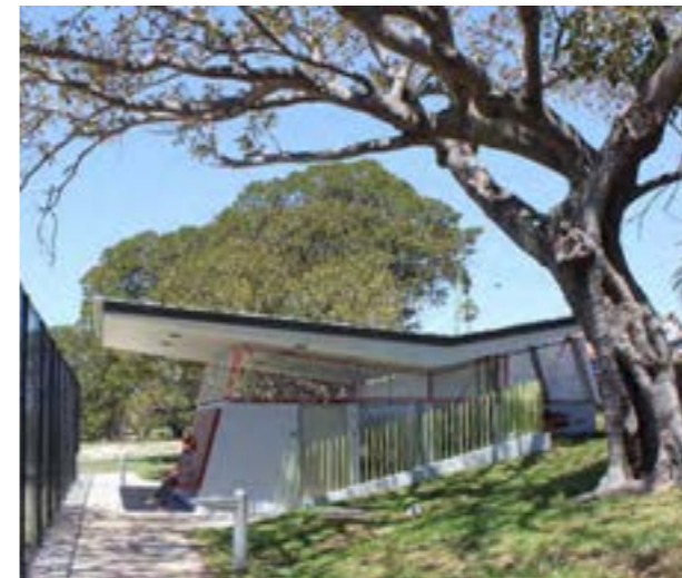
Baker Park amenities by Phillips Marler - single storey amenities building built into adjacent embankment
