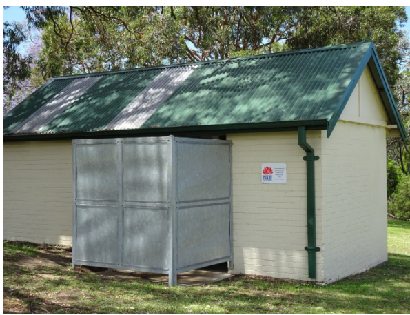
Toilets at Tygarah Park
