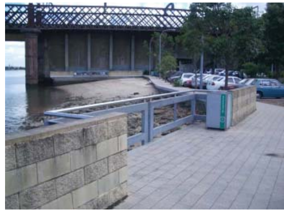
Lookout at Meadowbank Ferry wharf. Location for signage integration to balustrades.
