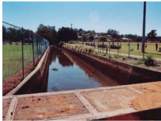
Stormwater channel in Meadowbank Park. Existing channel with potential to interpret changes in landform, water flow and ecology. Selective rehabilitation potential.
