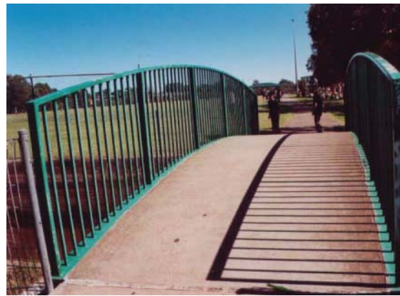
Bridge crossing channel in Meadowbank Park. Potential to link bridge into recreational loop paths. Modify handrail to include integrated artwork.
